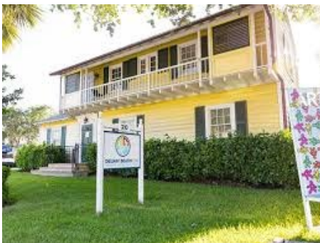
20 N Swinton Ave – CRA Office
