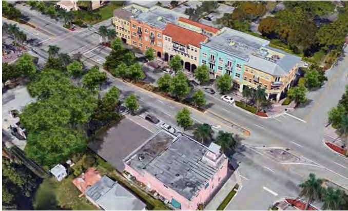
Existing West Atlantic Avenue
