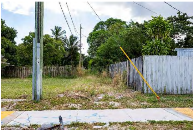
Deteriorating conditions in alleys
