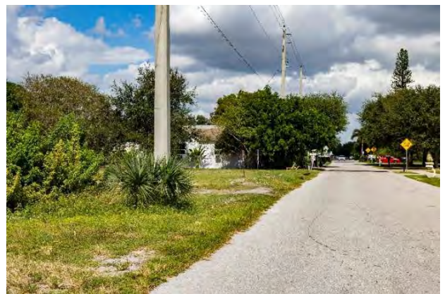
Lack of sidewalk on neighborhood streets
