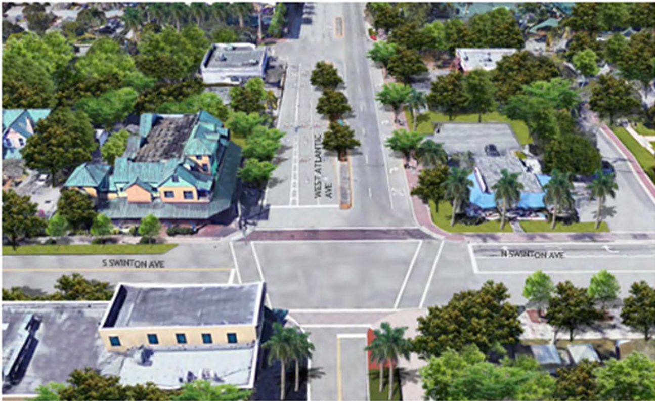
Existing Swinton Avenue and Atlantic Avenue Intersection
