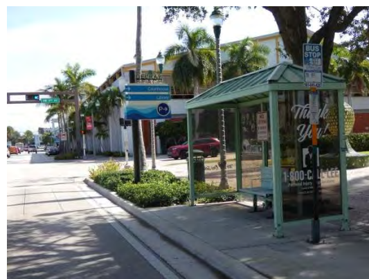
W. Atlantic Avenue Streetscape Improvement
