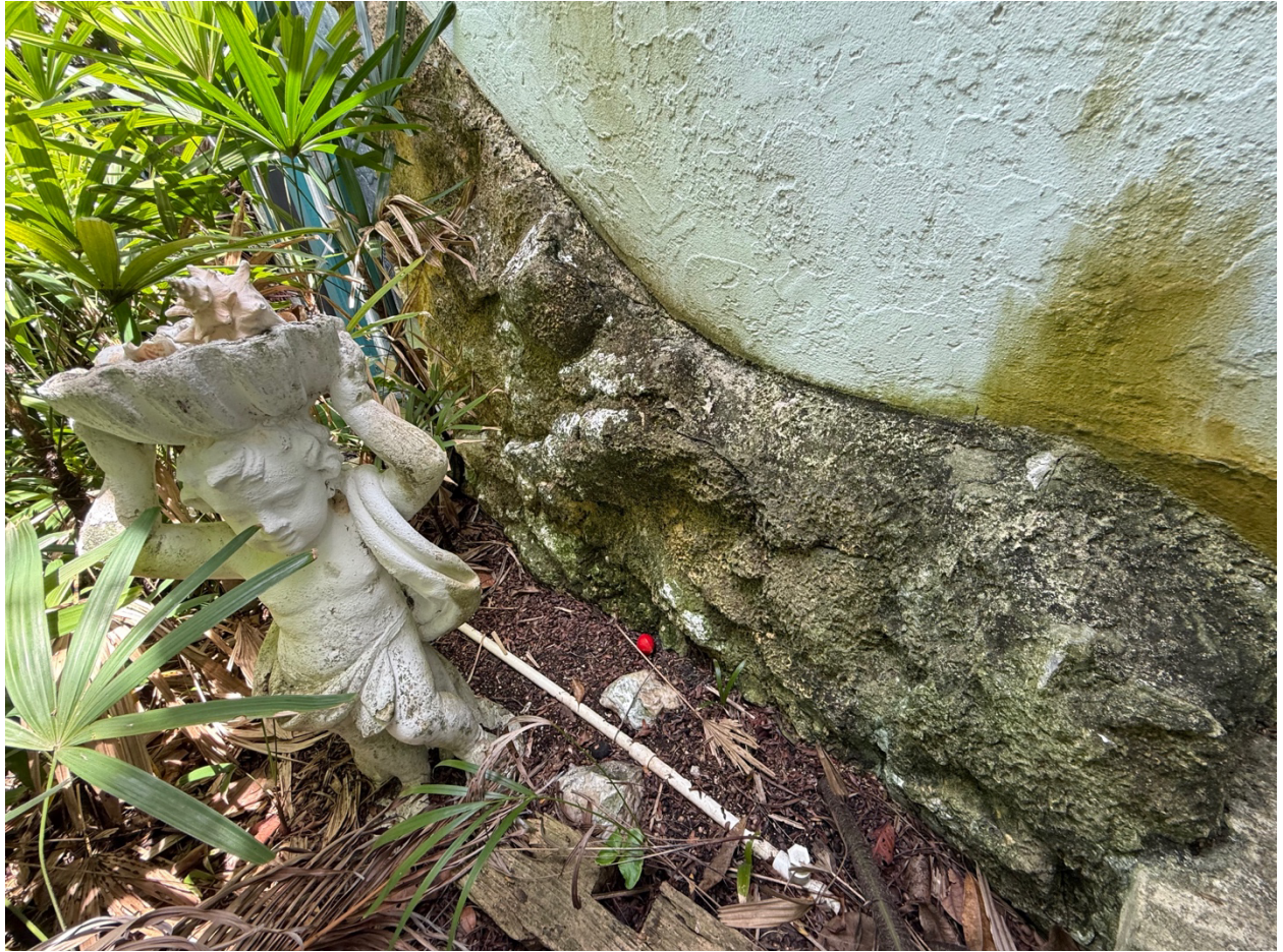
Current Existing Coral on North Elevation
