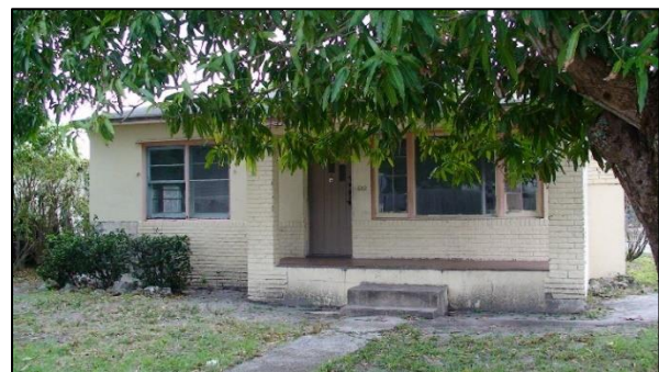
Abandoned Home in Delray Beach
