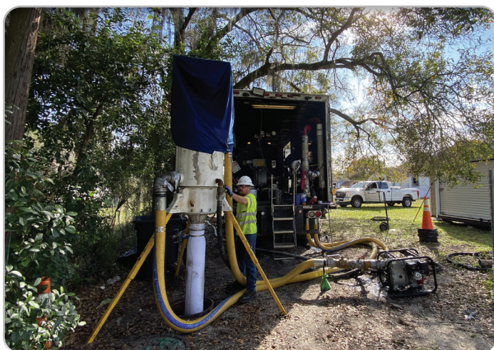
Lining Sanitary Mains in City Easements
