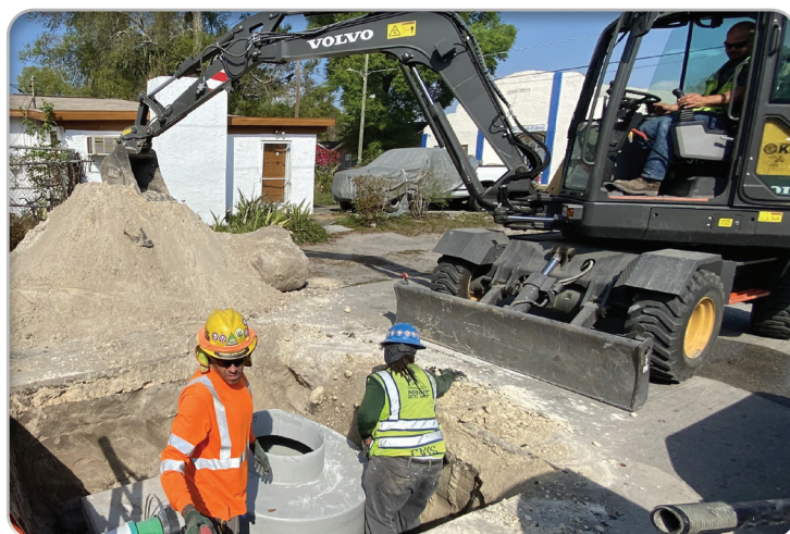
Installing New manholes at mainline terminations.
