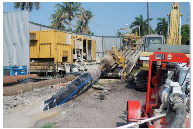
24-inch Water Main and 24-inch Force Main Subaqueous Pipeline Installations, City of West Palm Beach
