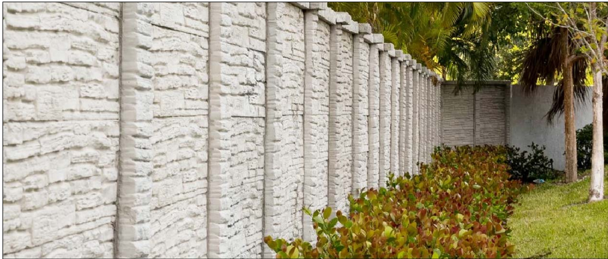
Typical View From Neighborhood Side Of Wall
