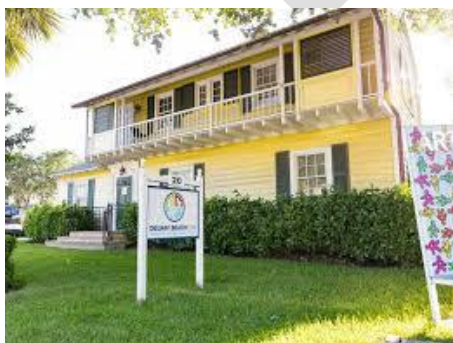
20 N Swinton Ave – CRA Office
