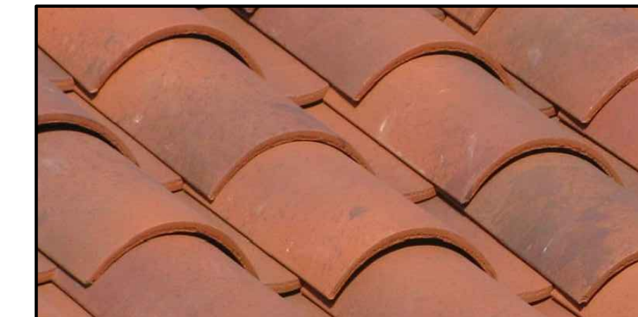
BARREL TILE TO MATCH EXISTING
