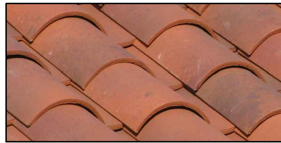
BARREL TILE TO MATCH EXISTING
