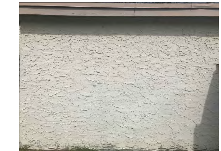
EXISTING STUCCO PATTERN
