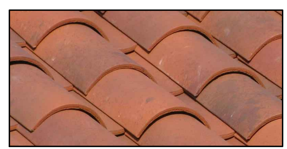
BARREL TILE TO MATCH EXISTING
