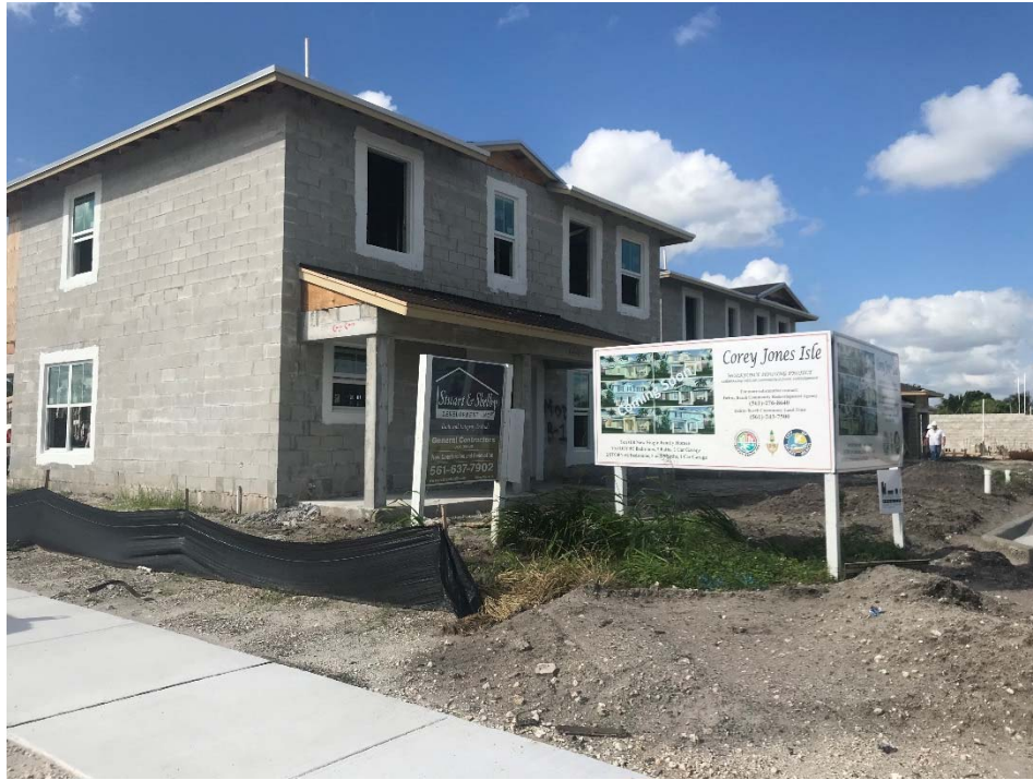
Photo 7: View of the Corey Jones residential development being constructed along the eastern side of SW 4 th Street.
