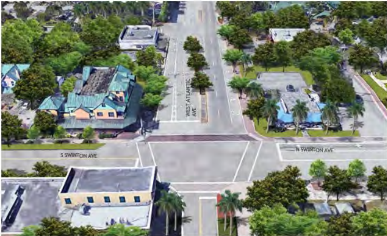
Existing Swinton Avenue and Atlantic Avenue Intersection
