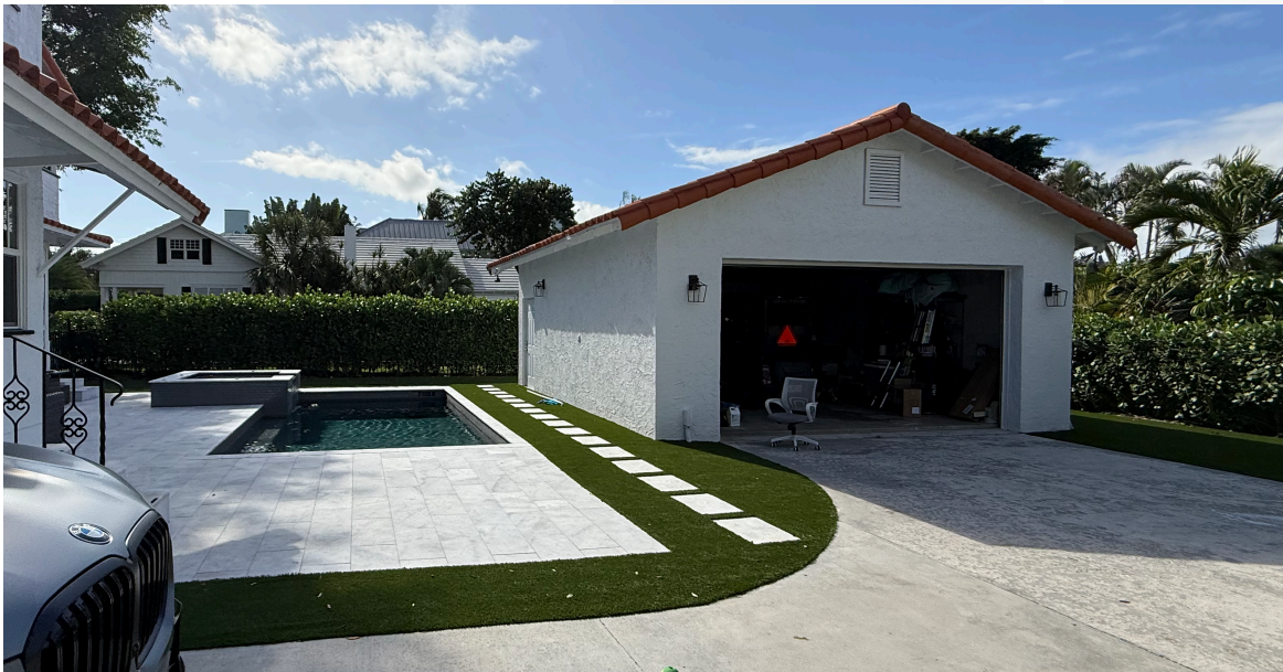
Existing (conditions of) detached Garage structure, in rear yard (west side of property)
