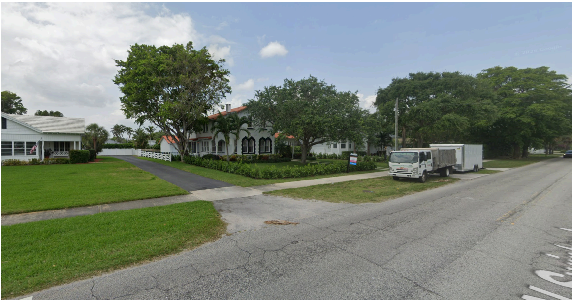
South view of exiting House from R.O.W.
