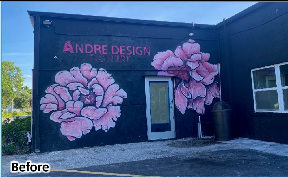
Building 1880 Façade 3 (File No. 2025-016)
