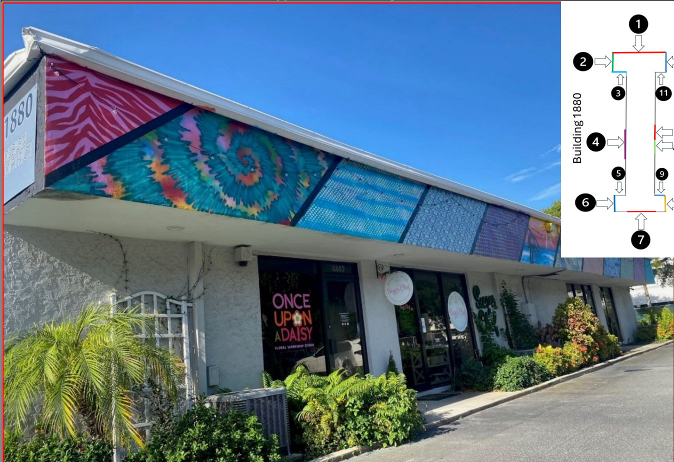
Building 1880 Façade 1 (File No. 2025-015) Approved on February 25, 2025
