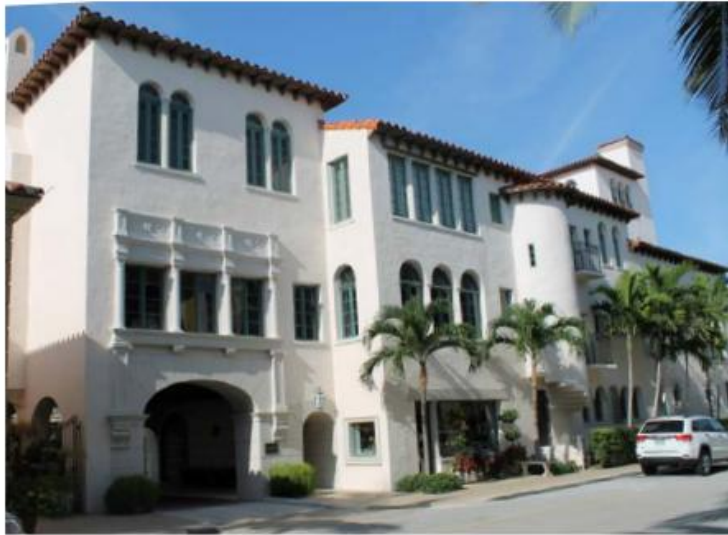
EVERGLADES CLUB, PALM BEACH, FL. This famous club was designed by architect Addison Mizner. The building extends along most of a city block, however, the composition of the massing is artfully broken up into smaller increments. The result is multiple building volumes providing a rich visual environment along the sidewalk and street.
