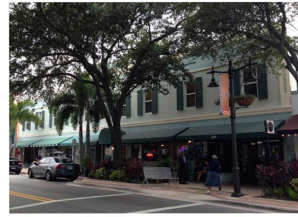
CLEMATIS CENTRE, WEST PALM BEACH, FL. This two-story building contains stores in the first story and residences in the second story. The facade is comprised of a series of storefronts and regularly spaced, vertically-proportioned windows with shutters in the second story.
