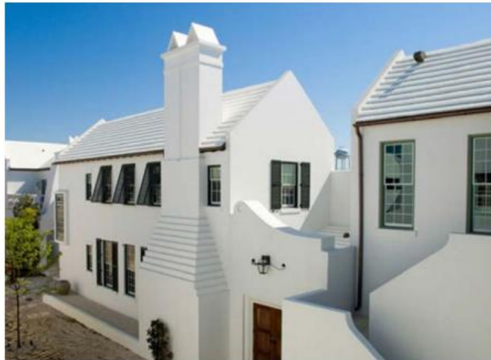
57 GOVERNORS COURT, ALYS BEACH, FL. Anglo-Caribbean architecture typically elaborates and sculptural shapes masonry elements. Generally this detailing occurs on the parapets, chimneys, entries, and stairways.
