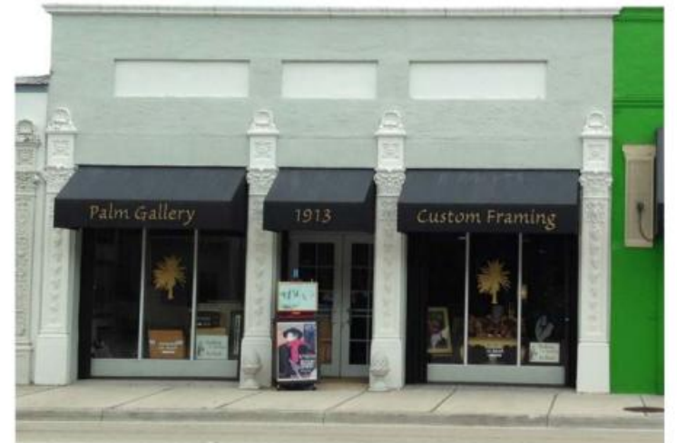
1913 S. DIXIE HIGHWAY, WEST PALM BEACH, FL. This shop illustrates the type of ornamental friezes and pilasters that were frequently incorporated in the 1920s. Buildings remain simple in form with decorative elements typically applied between bays, around openings, or within parapets.
