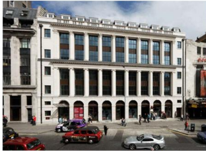
TOTTENHAM COURT ROAD, COMMERCIAL BUILDING, LONDON This recently constructed commercial building was designed by Quinlin Terry. The six-story building is cleverly disguised in a three-story composition. This play of scale maintains classical proportions while making the building appear smaller.
