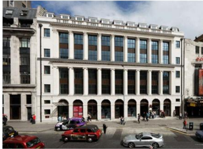
TOTTENHAM COURT ROAD, COMMERCIAL BUILDING, LONDON This recently constructed commercial building was designed by Quinlan Terry. The six-story building is cleverly disguised in a three-story composition. This play of scale maintains classical proportions while making the building appear smaller.
