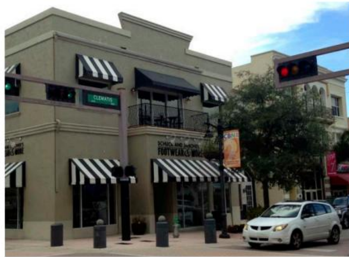
MIXED-USE BUILDING, WEST PALM BEACH, FL. This Main Street Vernacular example has a symmetrical facade comprised of three bays, with the center emphasizing entry to the store. Ornamentation is limited to a simple cornice line between the first and second stories and an articulated parapet. Shade is provided from awnings and street trees.
