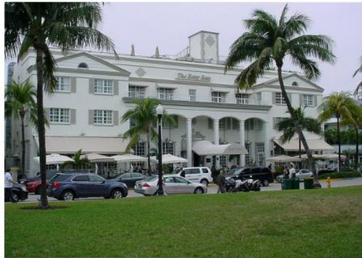
THE BETSY ROSS, MIAMI BEACH, FL This hotel has a classical, symmetrical facade with a double-height porch in the center flanked by volumes with simple gabled ends. Windows align in vertical pattern. The modest detailing is also consistent with Florida Vernacular architecture’s application of classical trim.
