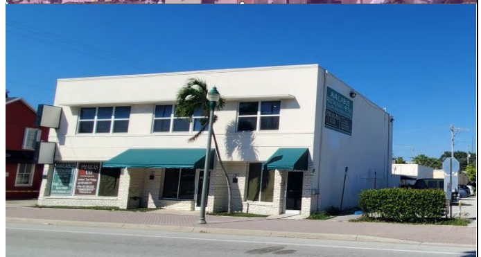
Existing Site Conditions
