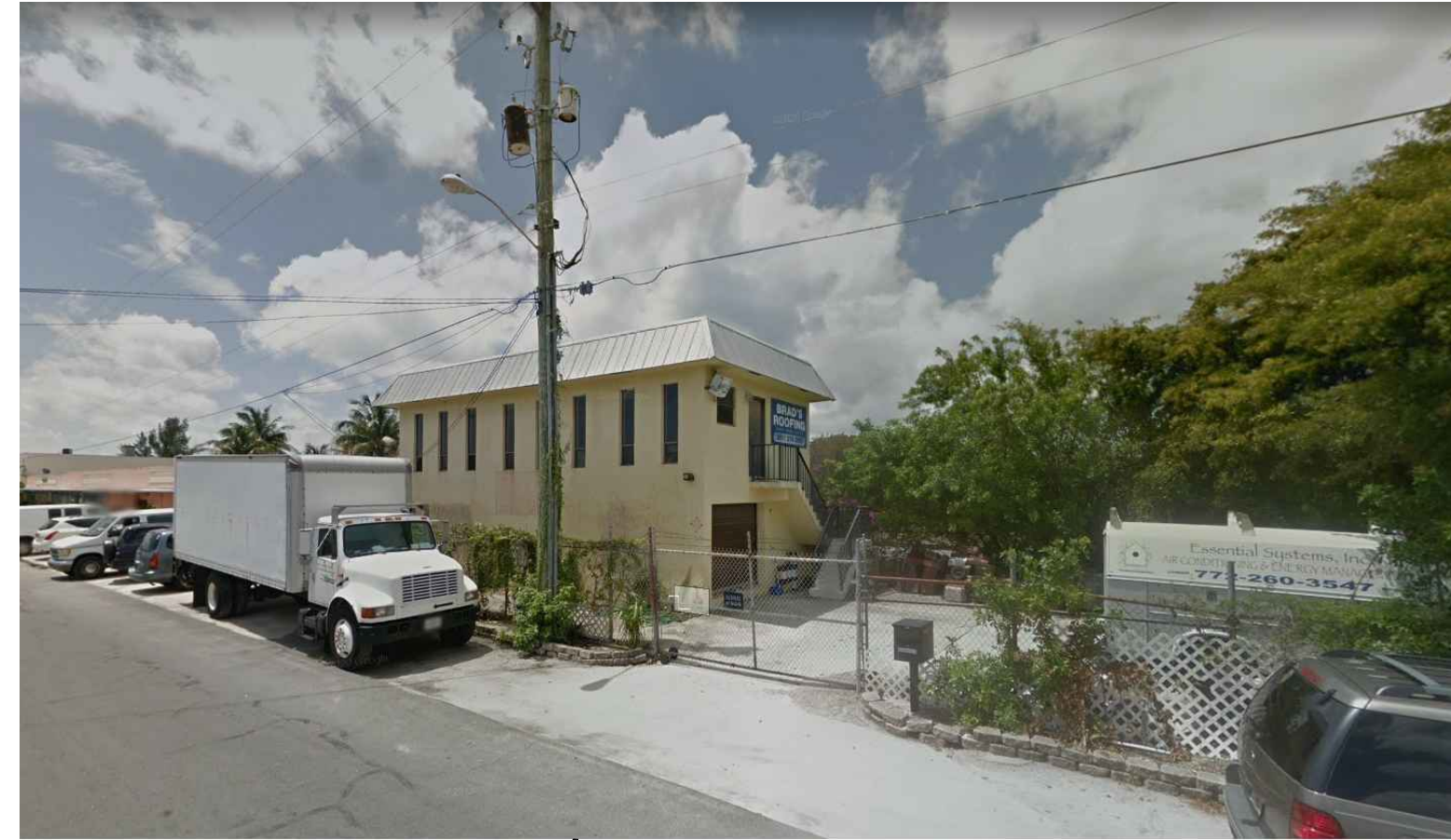
380 SE 2ND AVE. (FRONT FACADE)
