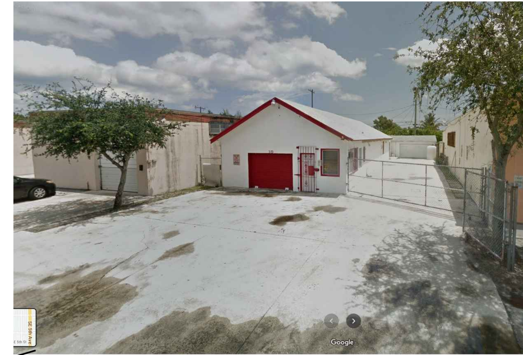
333 SE 2ND AVE. (FRONT FACADE)
