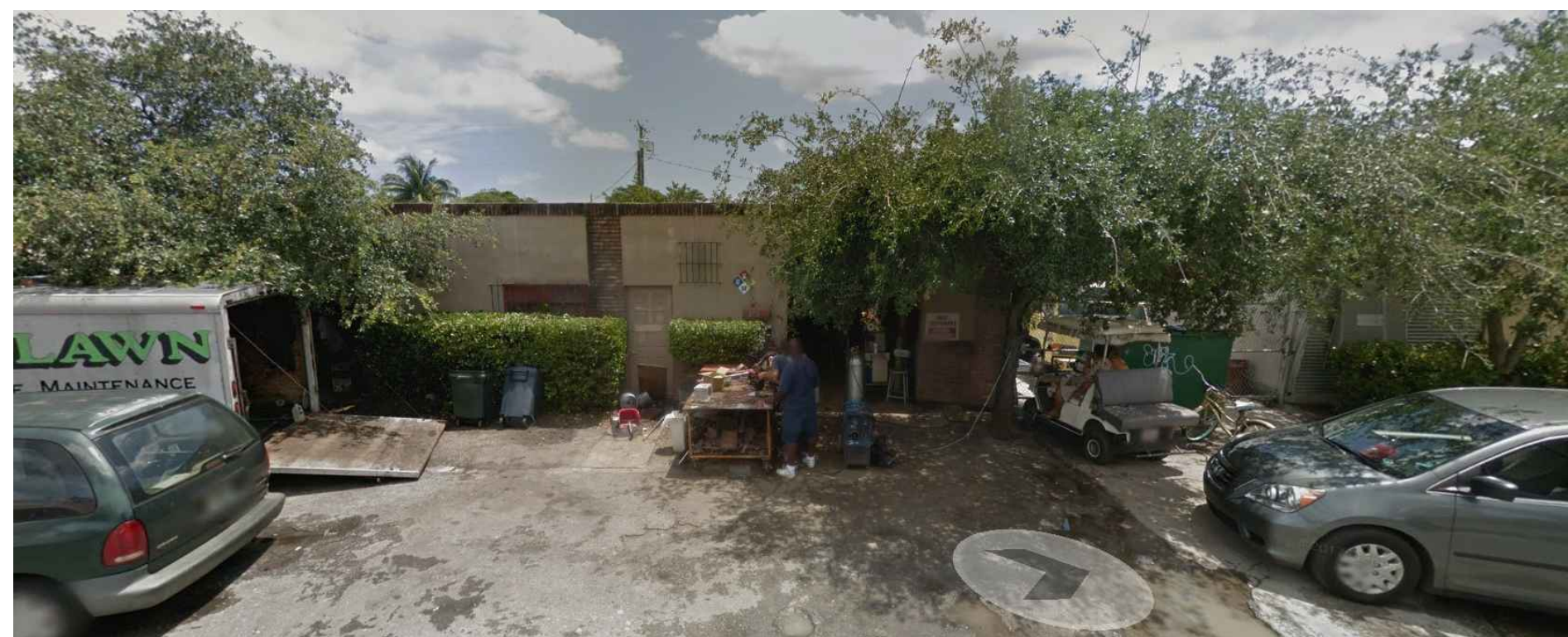
375 SE 2ND AVE. (FRONT FACADE)
