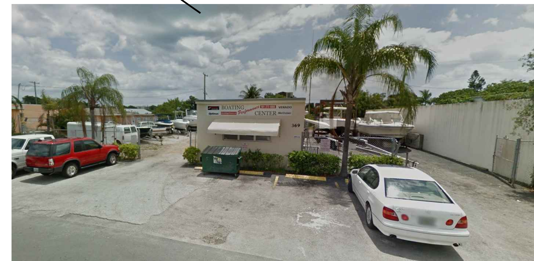
369 SE 2ND AVE. (FRONT FACADE)
