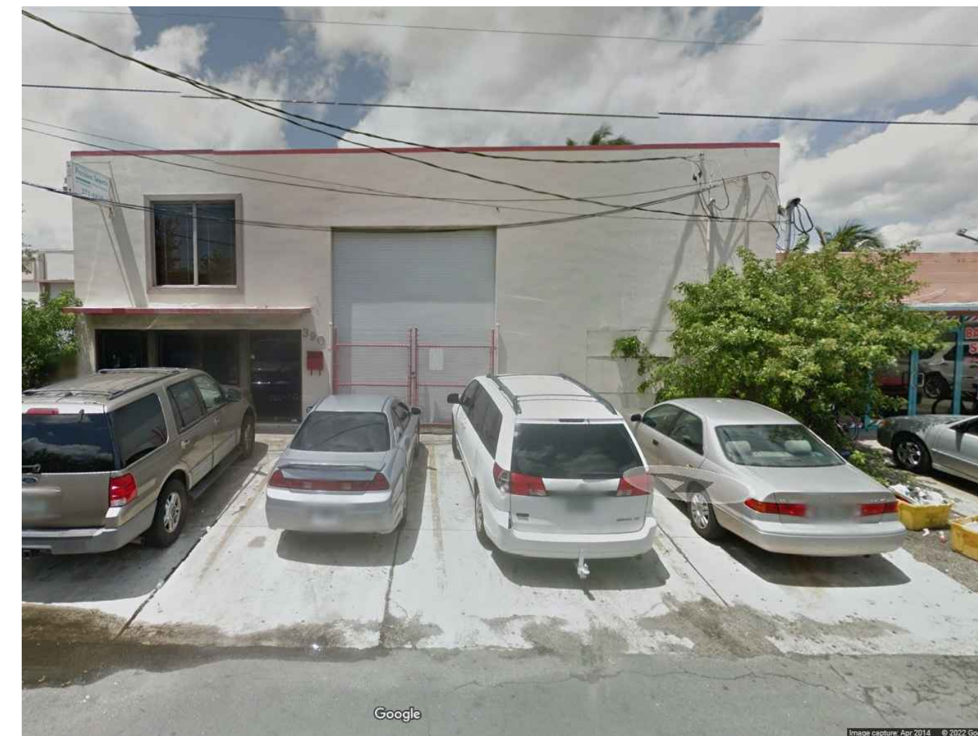
390 SE 2ND AVE. (FRONT FACADE)
