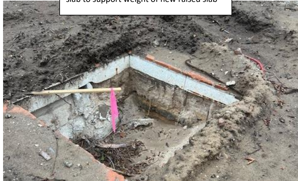
One of five Helical piles cut into existing slab to support weight of new raised slab
