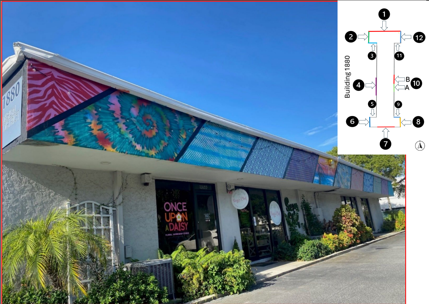
Building 1880 Façade 1 (File No. 2025-015)
