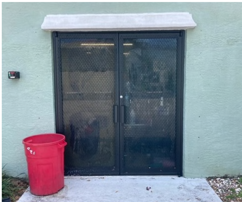
Image 10 Side Door Facing Right-of-Way
