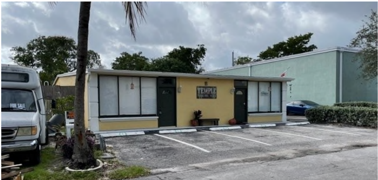
Image 2 Building Directly Behind Barkingham Palace
