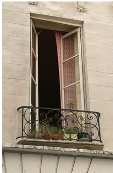
BALCONIES & RAILINGS. Decorative railings should be used on building facades when they serve a function such as on an occupiable balcony, enclosing planting areas, or as a safety measure for large windows in upper stories. Grills should not be applied to facades without serving a true function (left).
