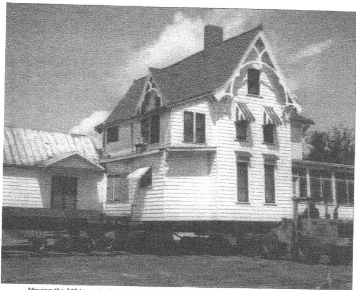
Moving the 240 tons structure required a 180 degree spin and a 90 degree turn.
