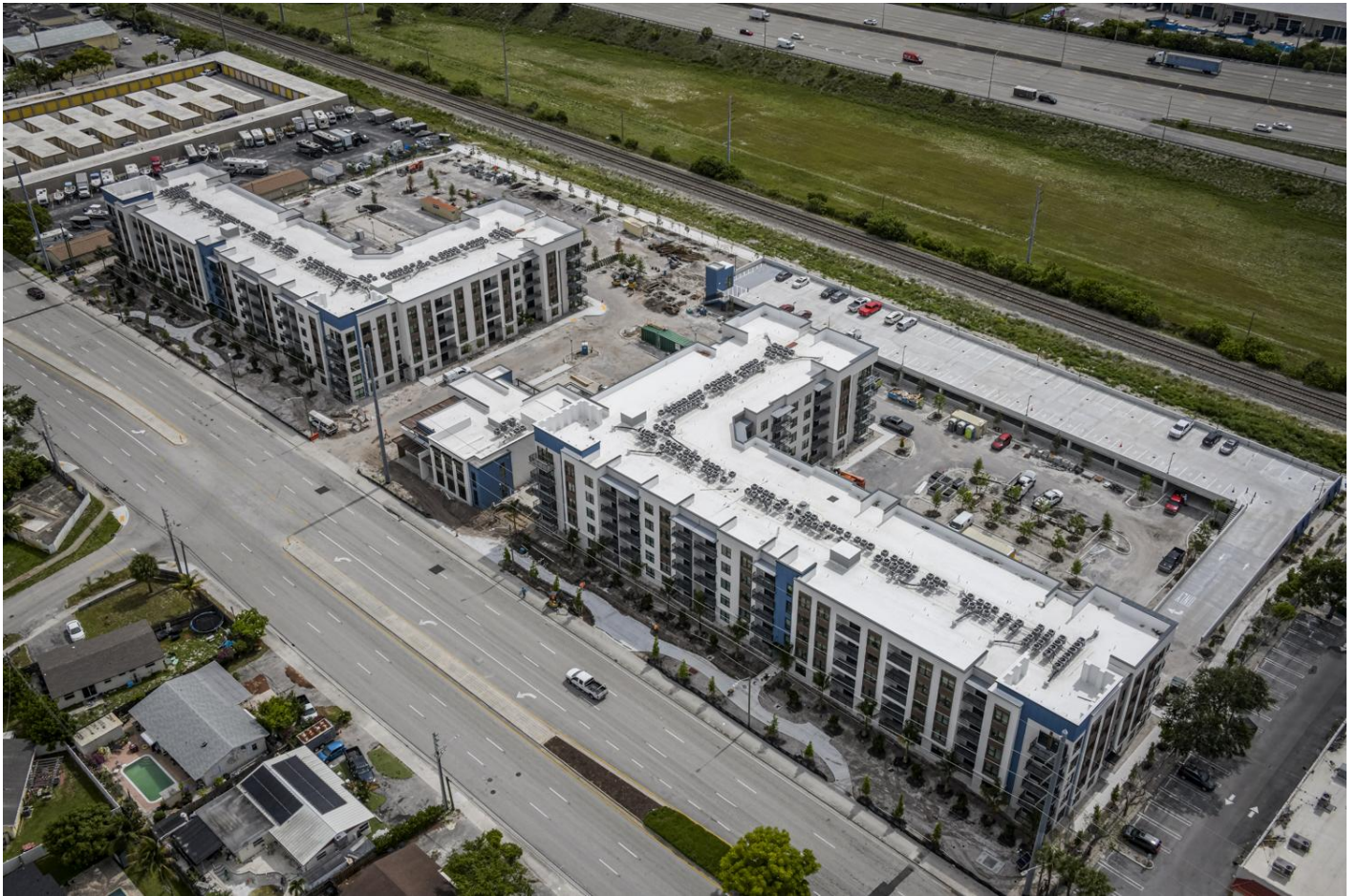
Overall Site Aerial (SW from Congress Ave.)
