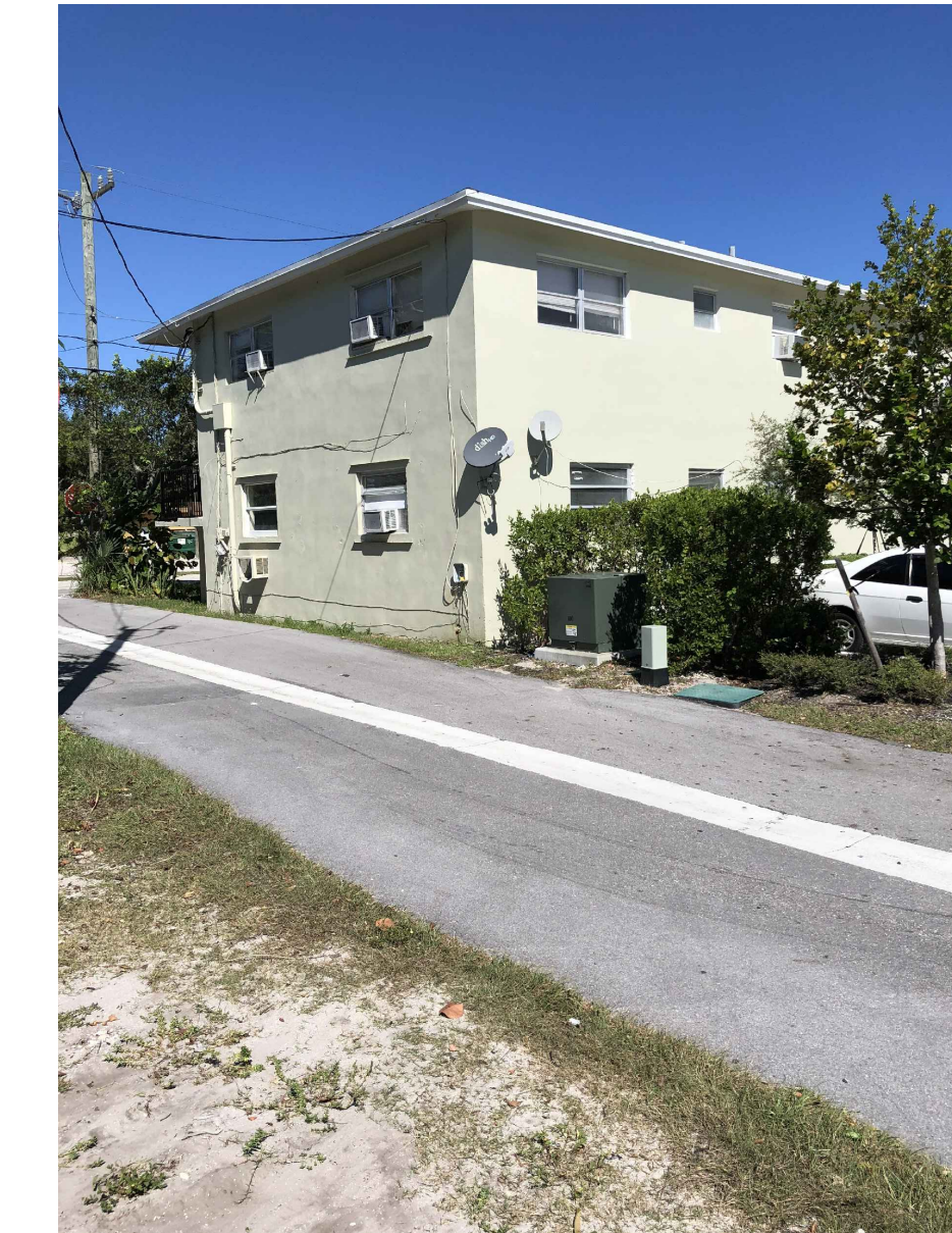
2 EXISTING WEST ELEVATION (LOOKING NORHTEAST)
