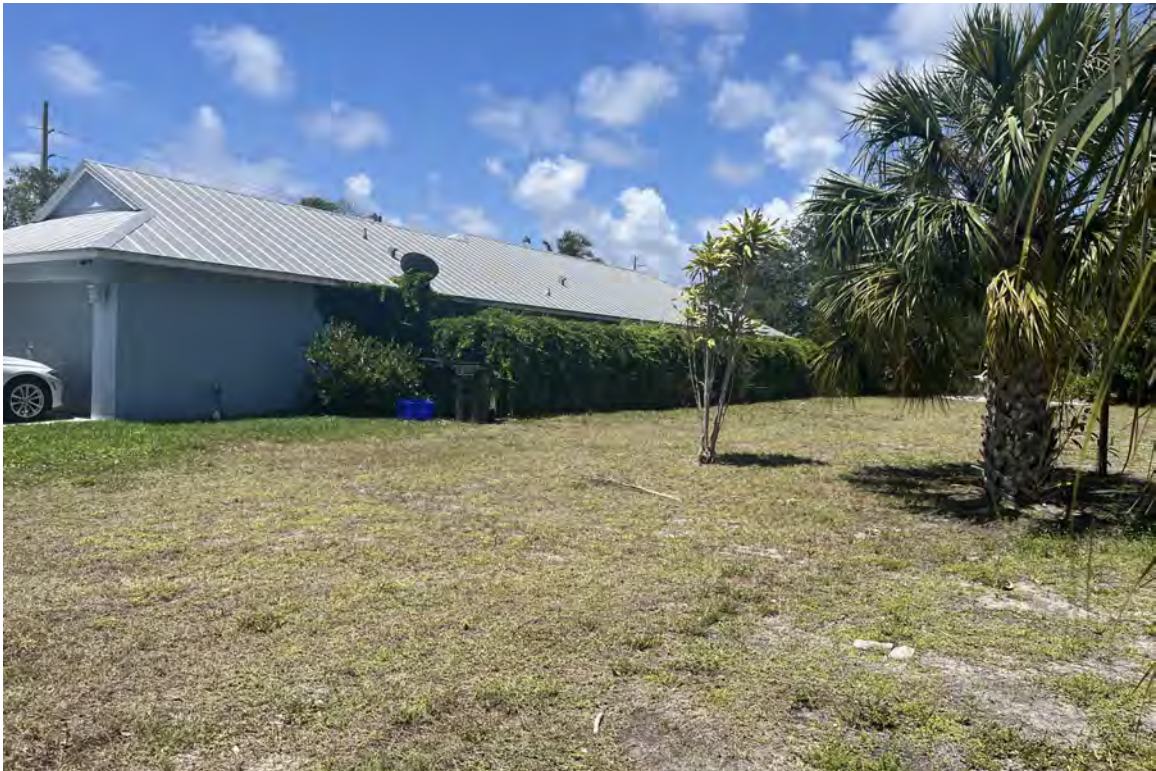
Overview from Northeast Corner
