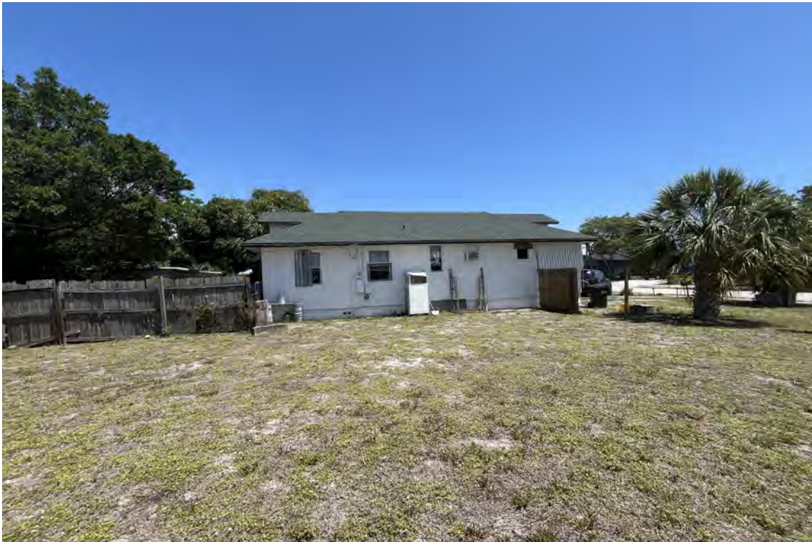
View north of the subject site
