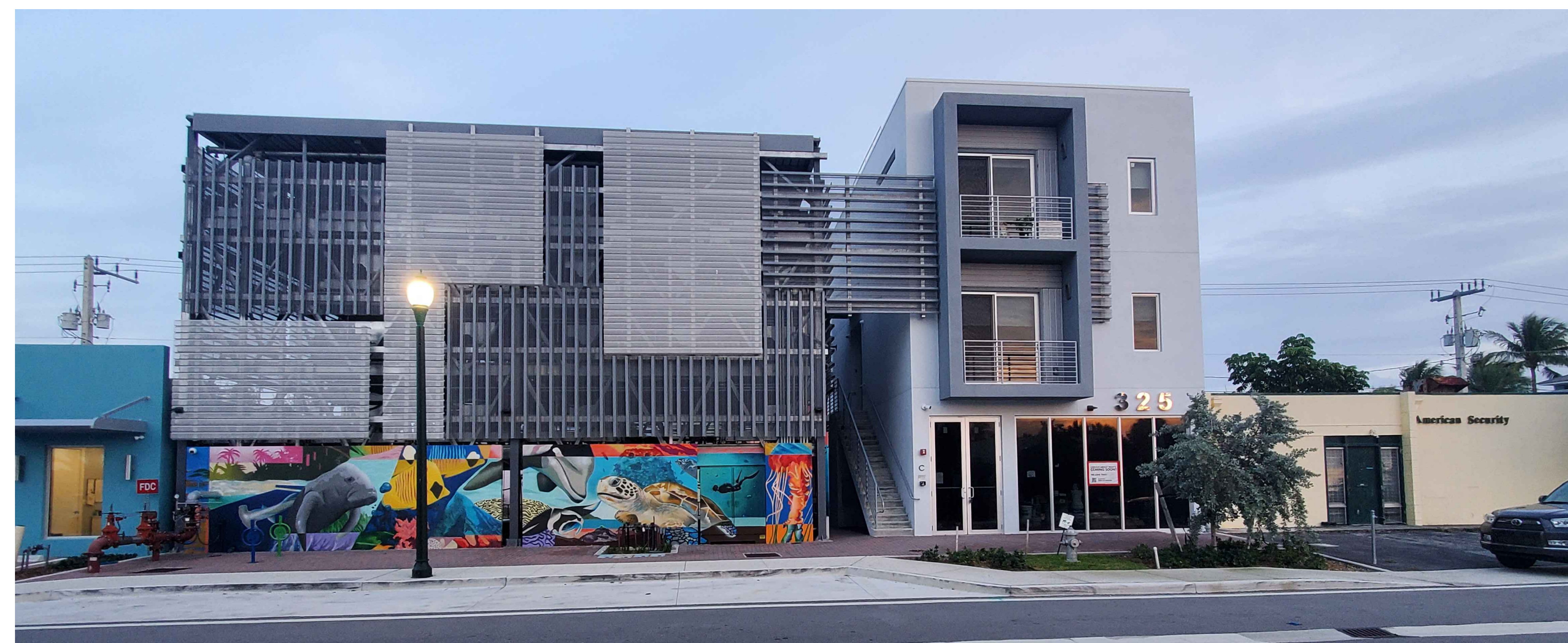
EXIST. BLDG. PHOTOGRAPH C SCALE N.T.S.
