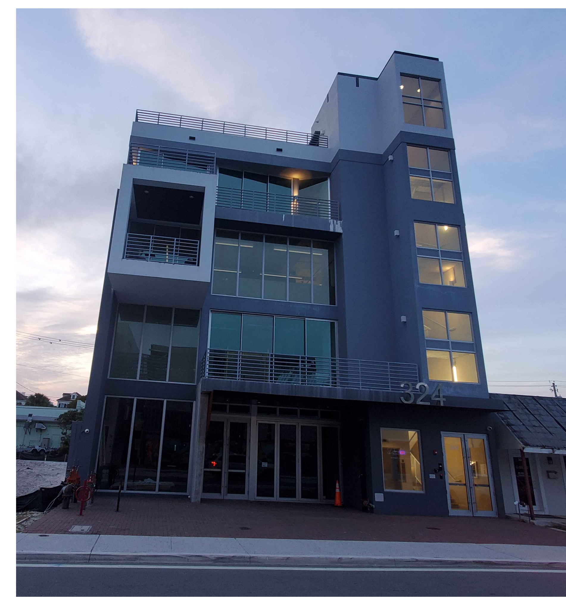
EXIST. BLDG. PHOTOGRAPH A SCALE N.T.S.
