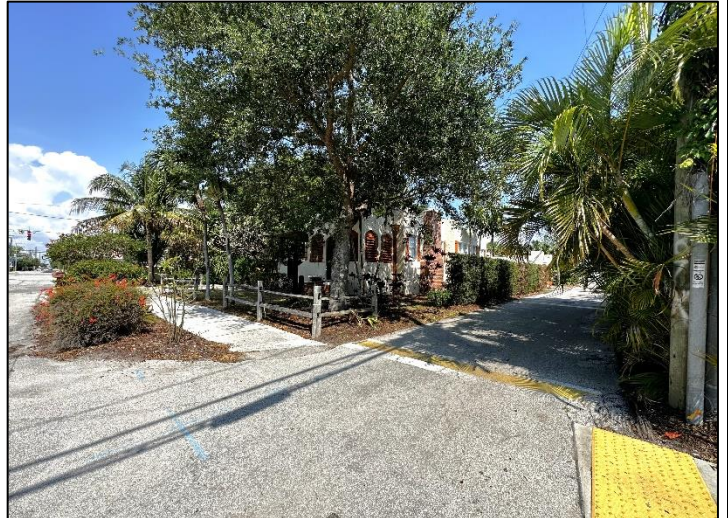
Residential building on the corner of NE 2 nd Street and the alley
