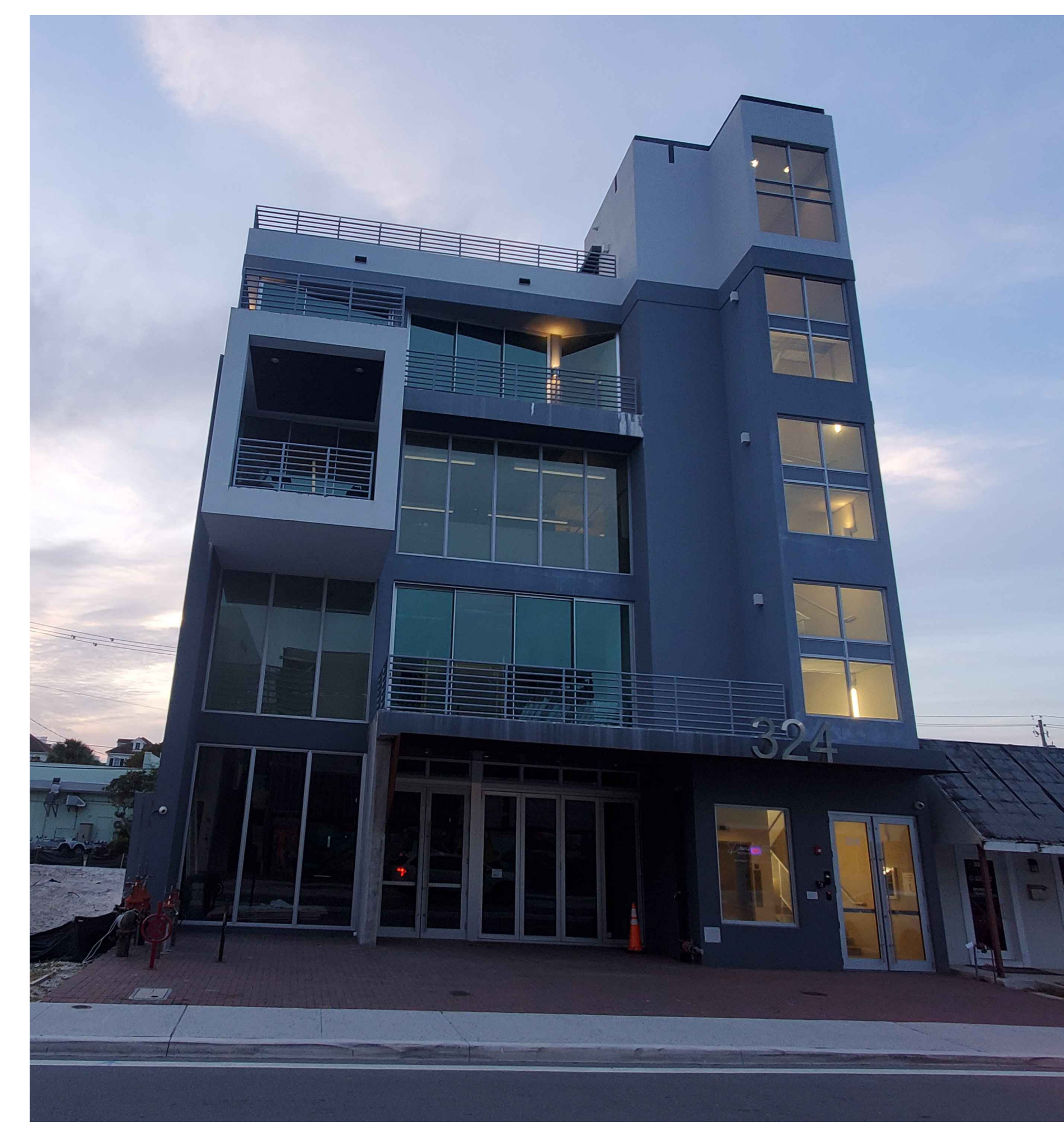
EXIST. BLDG. PHOTOGRAPH A SCALE N.T.S.
