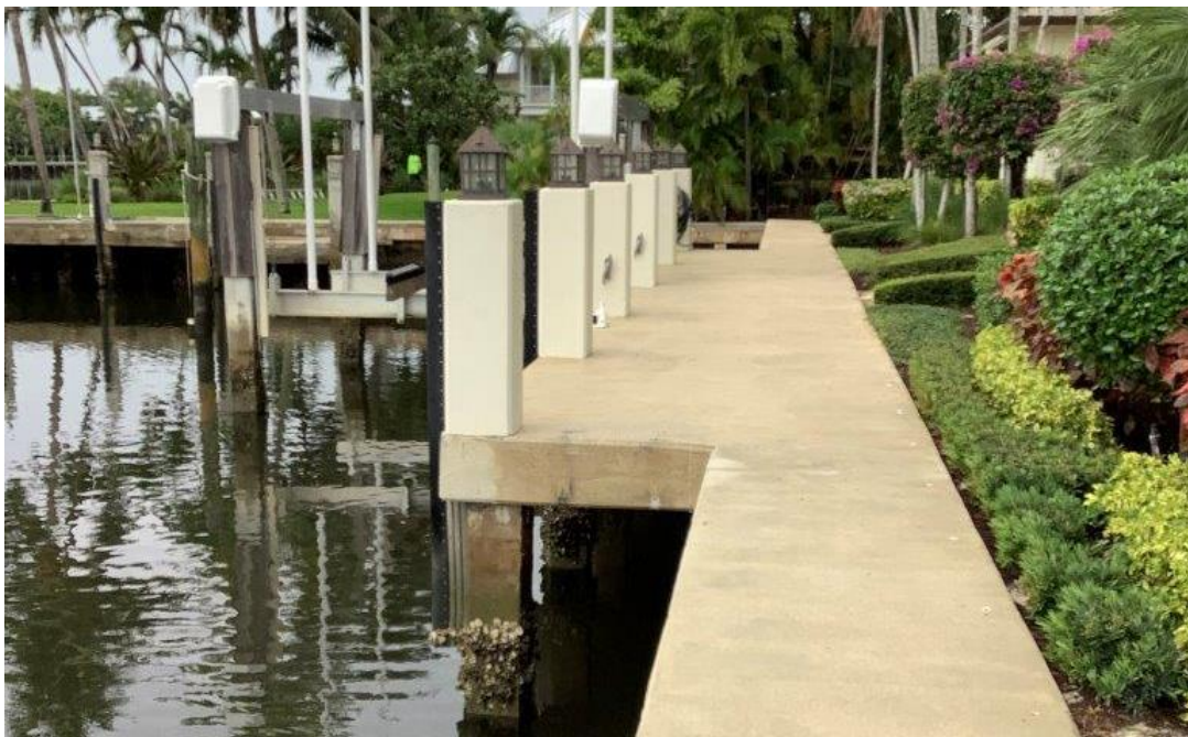
Existing Boat Lift & Marginal Dock
