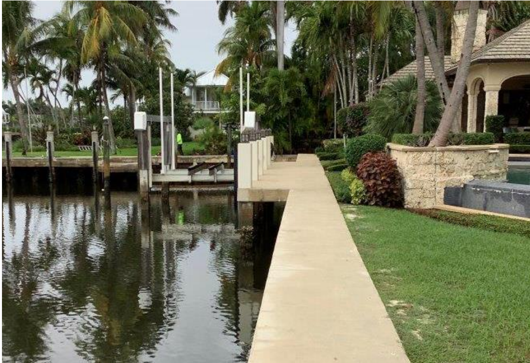
Existing Boat Lift & Marginal Dock
