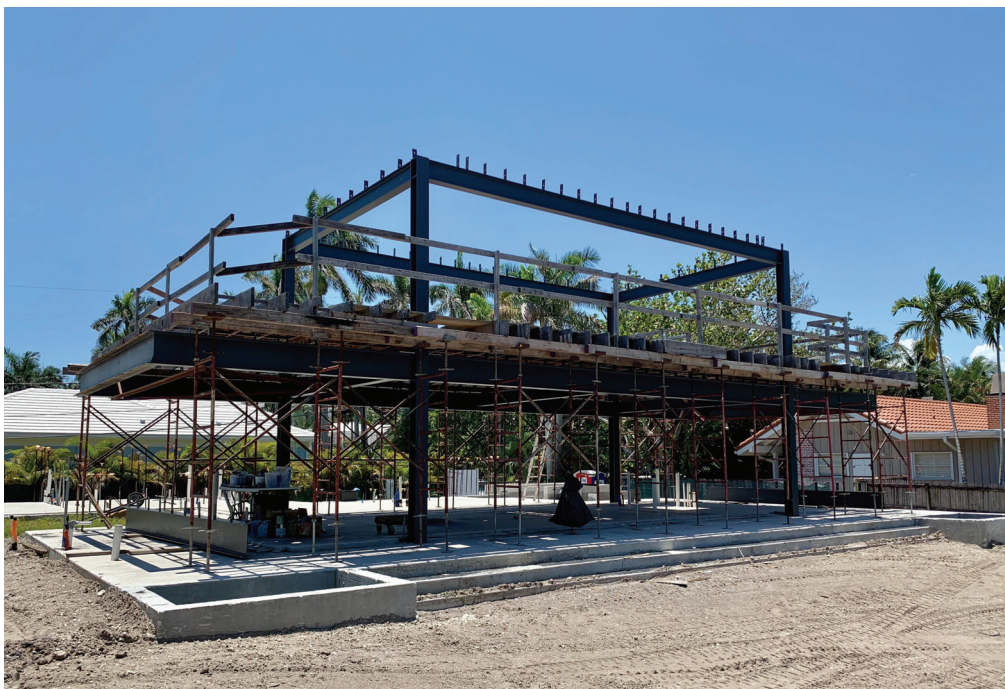
EXISTING STRUCTURE AFTER ELEV CHANGE, DEMO & STEEL PRESERVATION MAY 5, 2021
