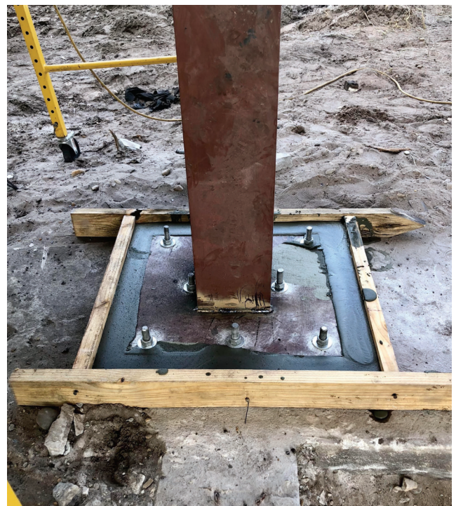
NEW STEEL PILE CAP PLATE & COLUMN SECTION MARCH 11, 2020
