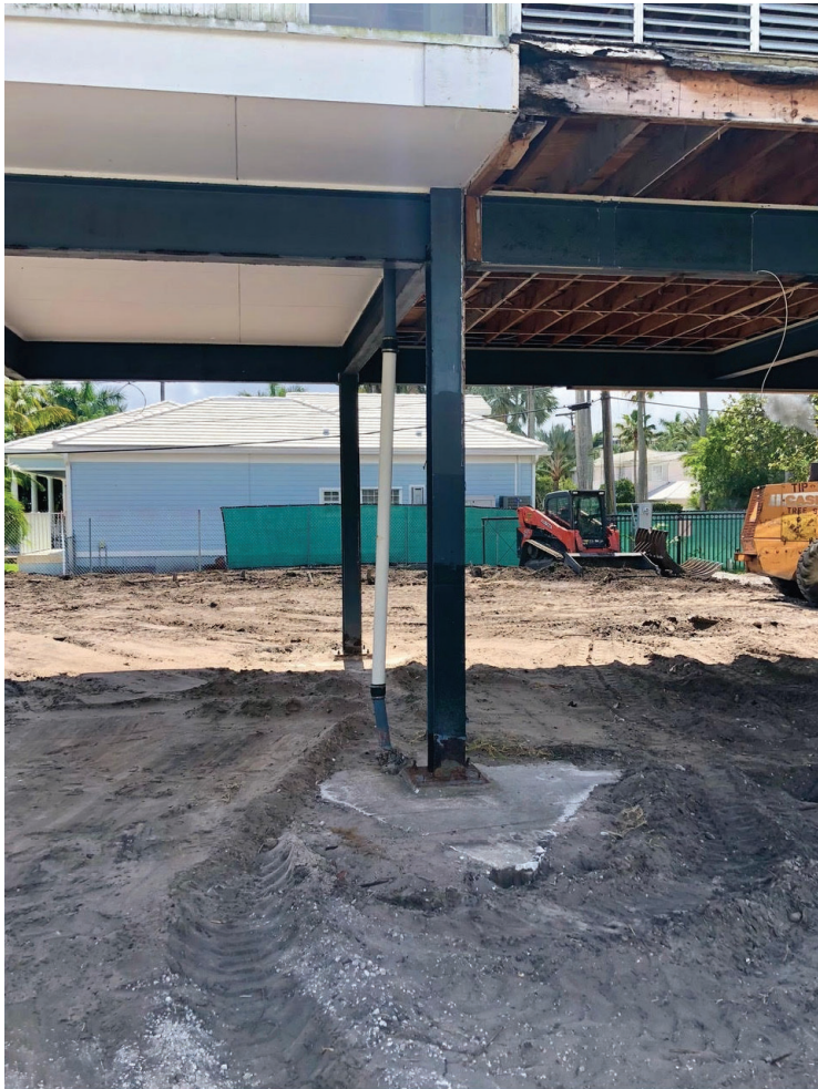
CORRODED STEEL COLUMN EXPOSED FEB 28, 2020
