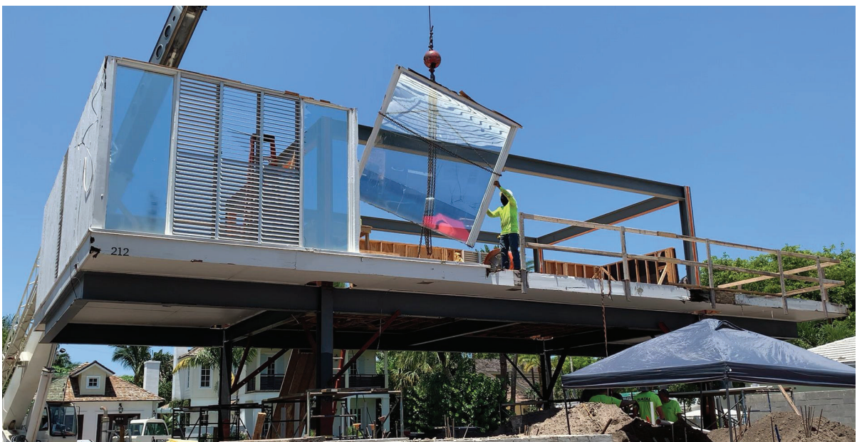
SEABREEZE SIDE EXISTING GLASS REMOVAL JULY 15, 2020 1:58 PM
