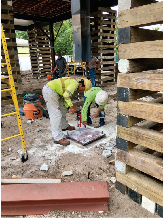
REPLACE STEEL COLUMN SECTION & PILE CAP PLATE MARCH 11, 2020
