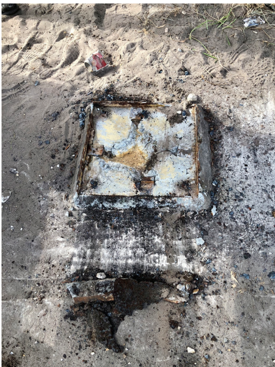
CORRODED STEEL PILE CAP PLATE MARCH 11, 2020
