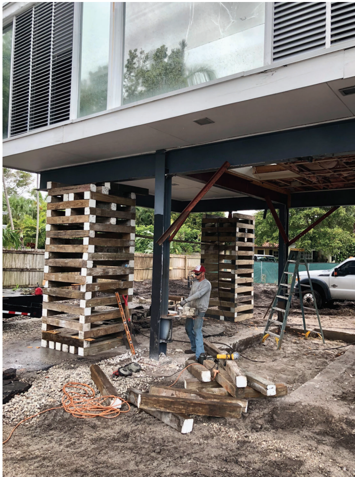
CUTTING OUT CORRODED STEEL MARCH 10, 2020
