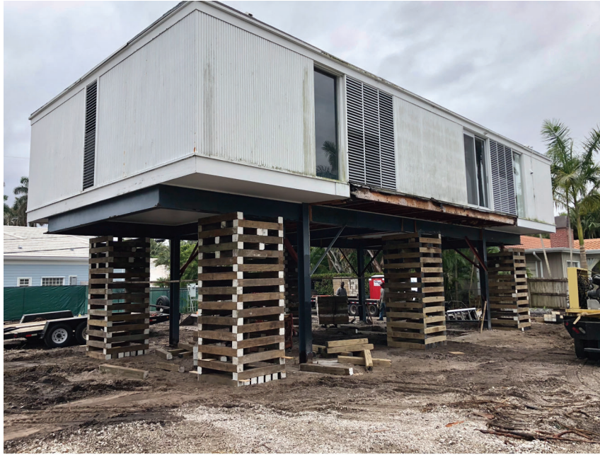
CRIBBING TO SUPPORT HOUSE DURING STEEL REPAIR MARCH 10, 2020
