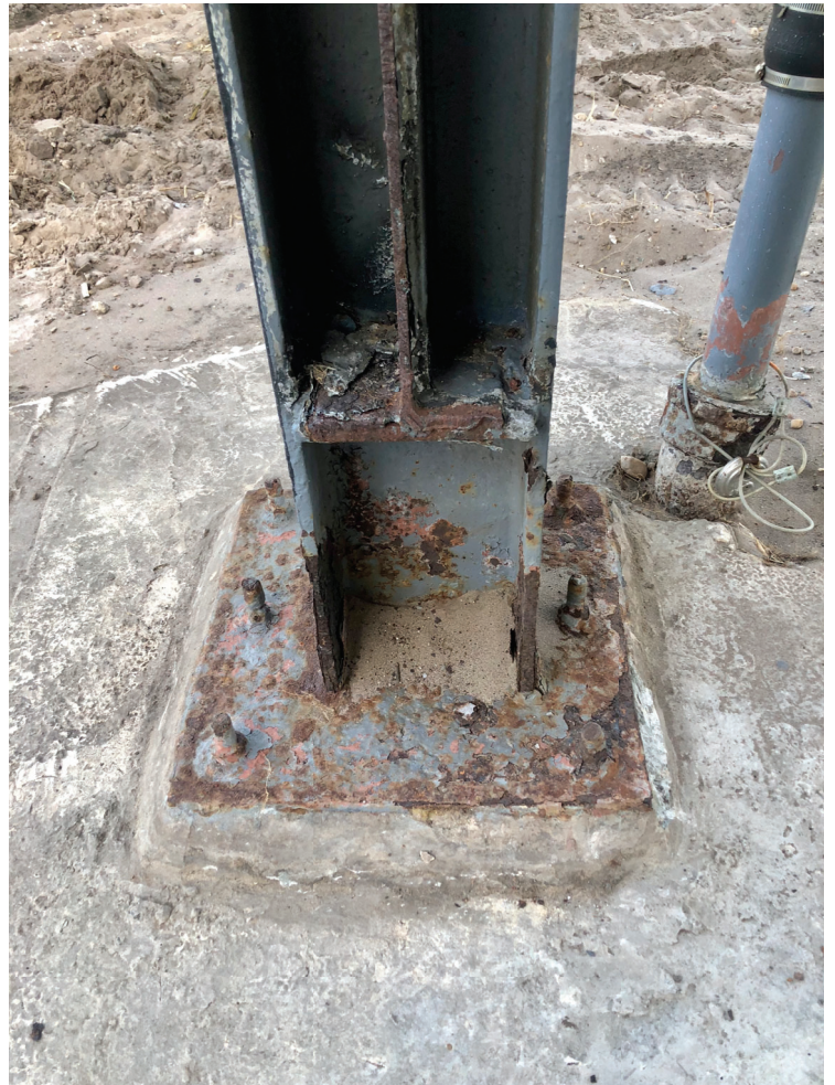
CORRODED STEEL COLUMN AND PLATE MARCH 5, 2020
