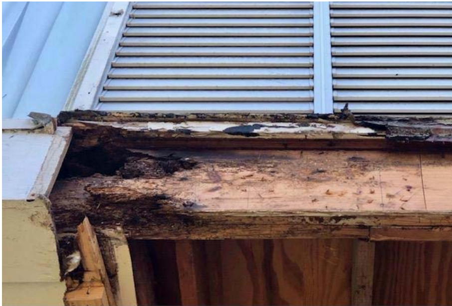
EXISTING 2ND FLOOR WOOD DAMAGE
