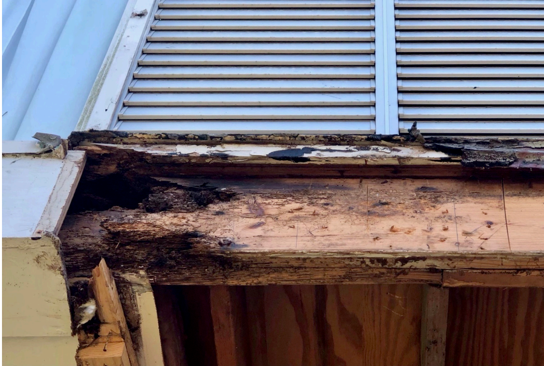
EXISTING 2ND FLOOR WOOD ROT JANUARY 15, 2019
