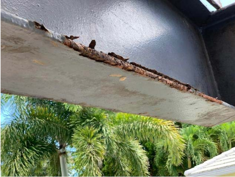
STEEL BEAM CORROSION
