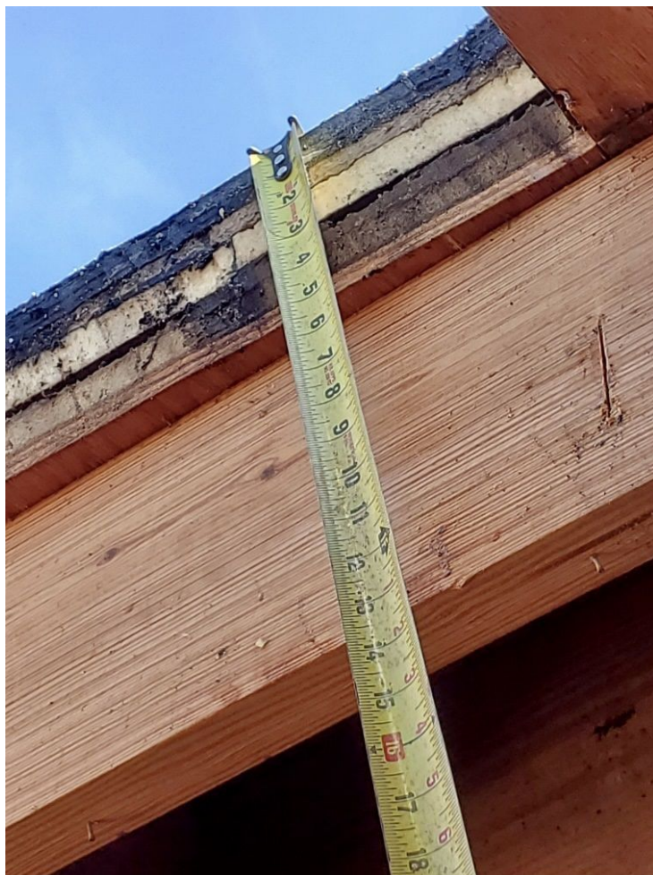
EXISTING 4 LAYER ROOF BEFORE REMOVAL
