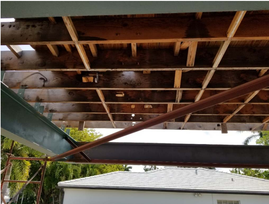
Exhibit 4. General view of Damaged Floor System oversized bored holes and notches
