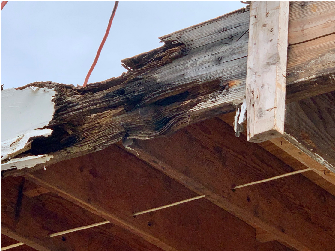
EXISTING ROTTEN WOOD 2ND FLOOR JULY 21, 2020
