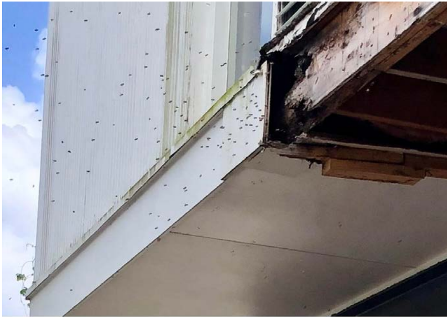
DAMAGE TO 2ND FLOOR WOOD DUE TO TERMITES/INSECTS
