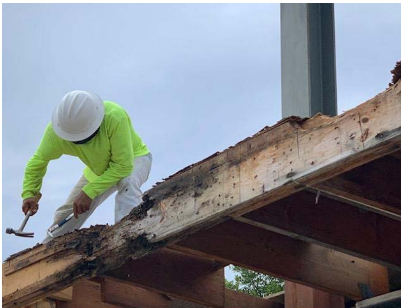
EXTENSIVE WOOD DAMAGE 2ND FLOOR
