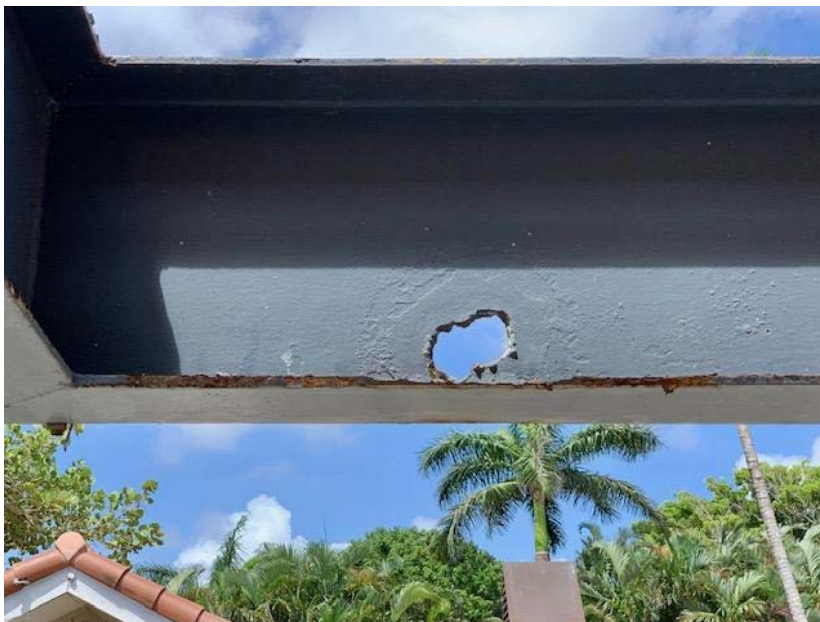
EXISTING STEEL BEAM DAMAGE
