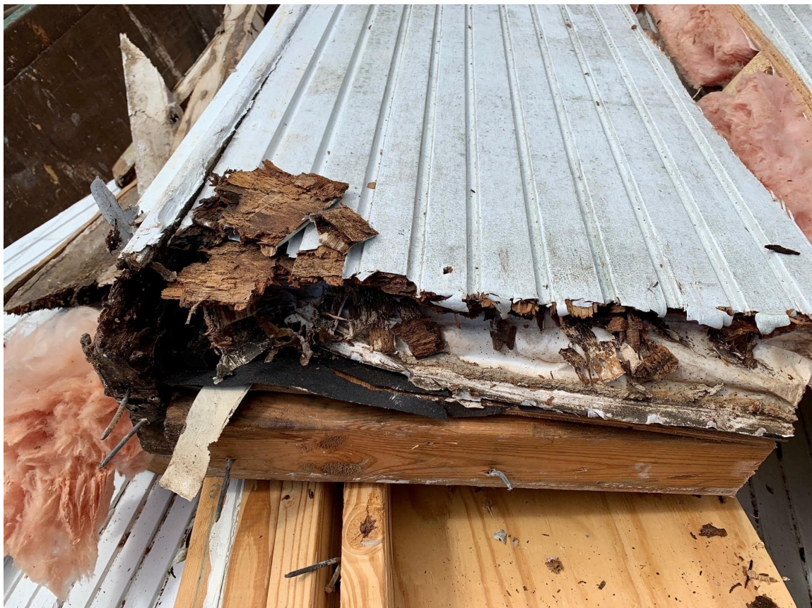
EXISTING ROTTED PLYWOOD SIDING JULY 20, 2020
