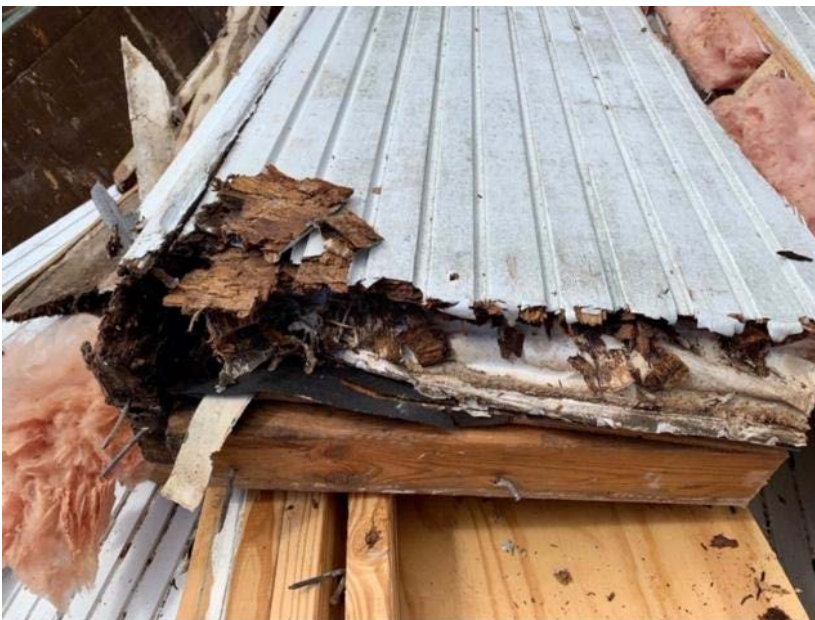
EXISTING ROTTED PLYWOOD SIDING
