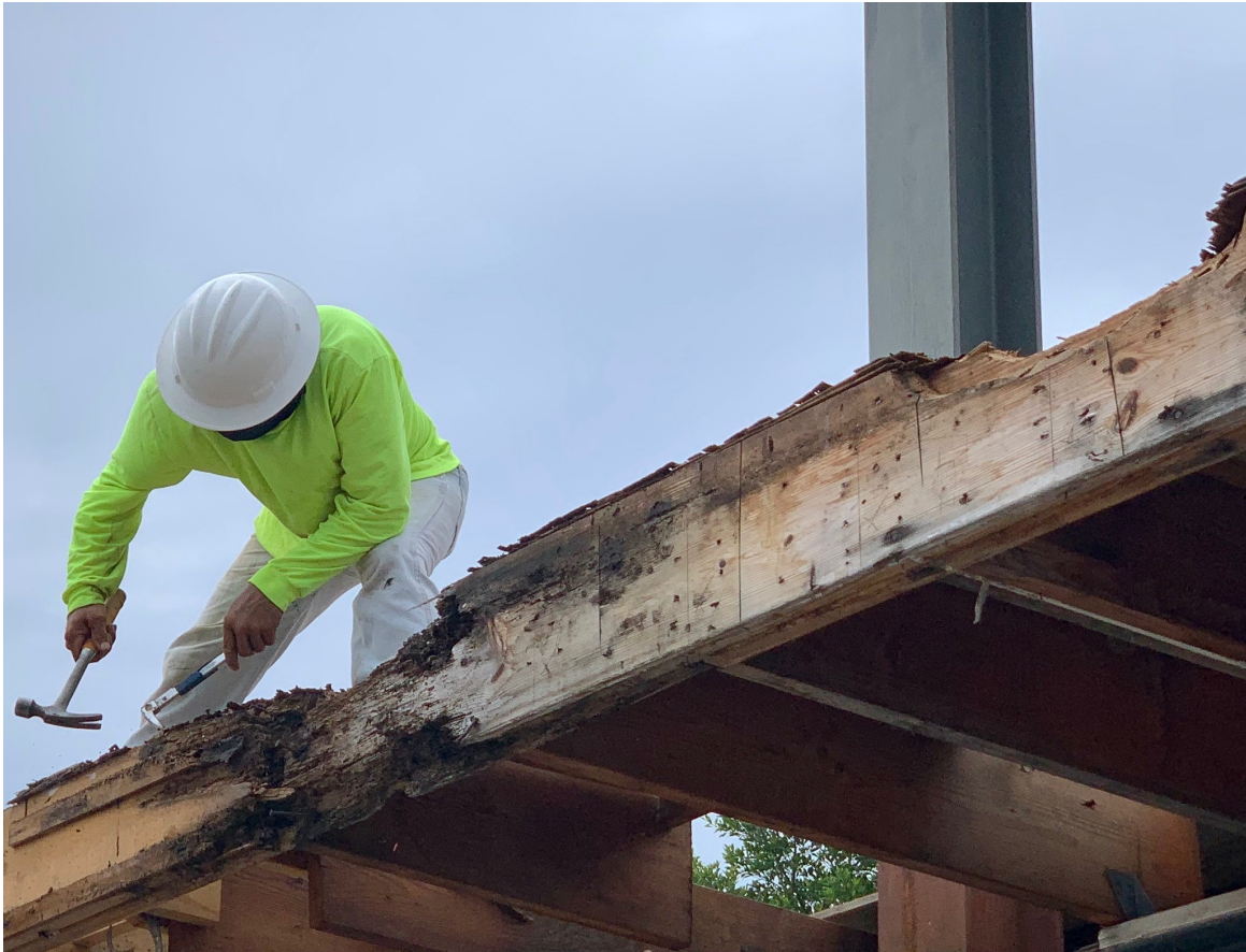
EXTENSIVE WOOD DAMAGE 2ND FLOOR JULY 21, 2020
