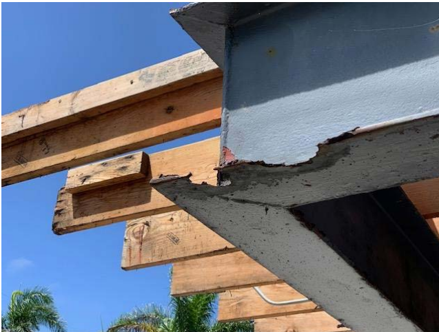
STEEL BEAM CORROSION
