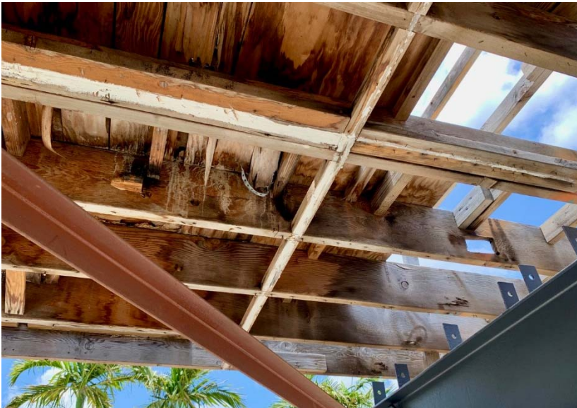
Exhibit 6. General view of Damaged Floor System
