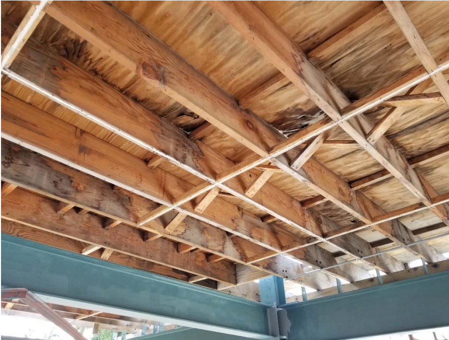
Exhibit 1. General view of Damaged Floor System
