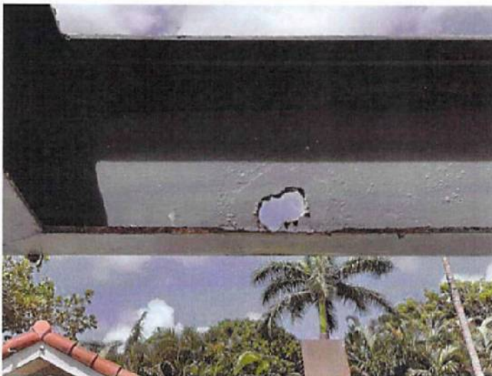
EXISTING STEEL BEAM DAMAGE
