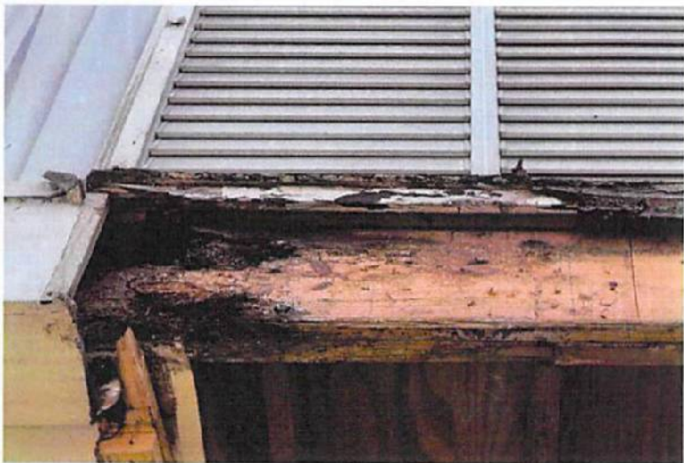
EXISTING 2ND FLOOR WOOD DAMAGE
