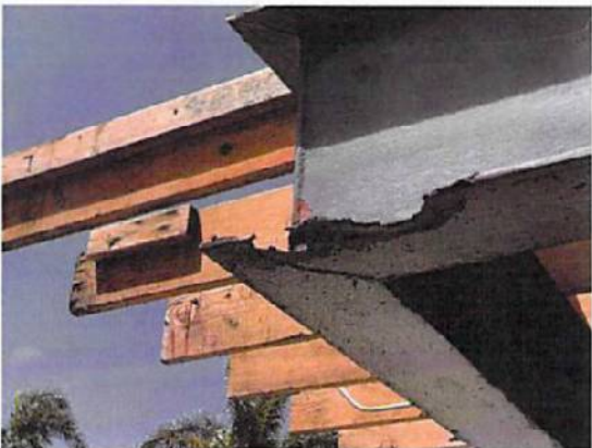
STEEL BEAM CORROSION
