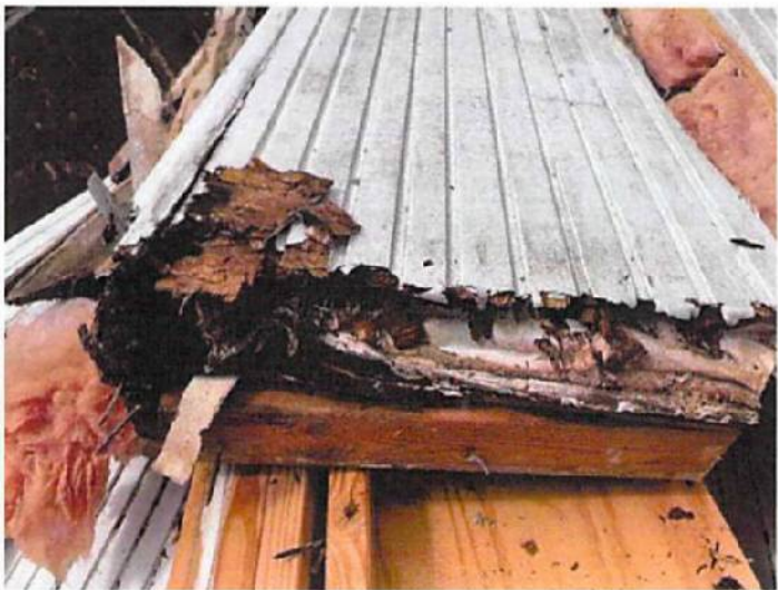
EXISTING ROTTED PLYWOOD SIDING
