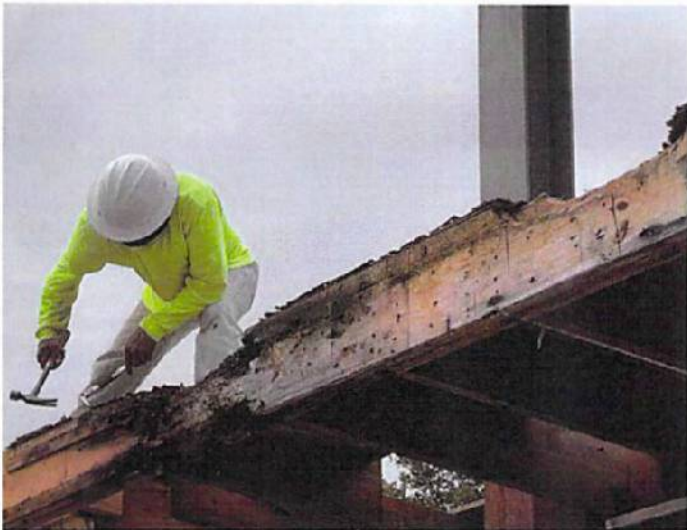
EXTENSIVE WOOD DAMAGE 2ND FLOOR
