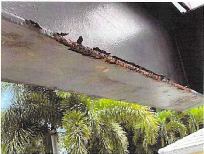
STEEL BEAM CORROSION
