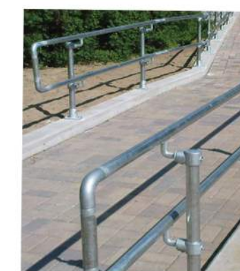
Galvanized Pipe Railing
