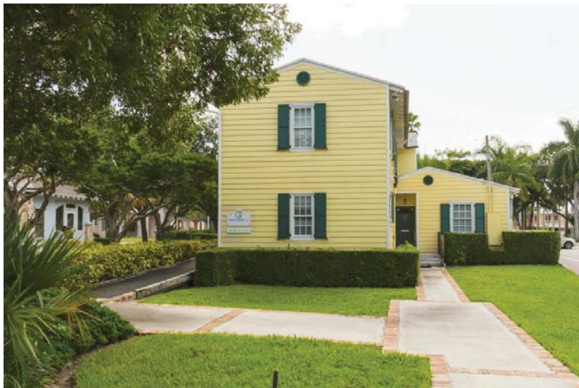
EXTERIOR ELEVATION - WEST FACADE
