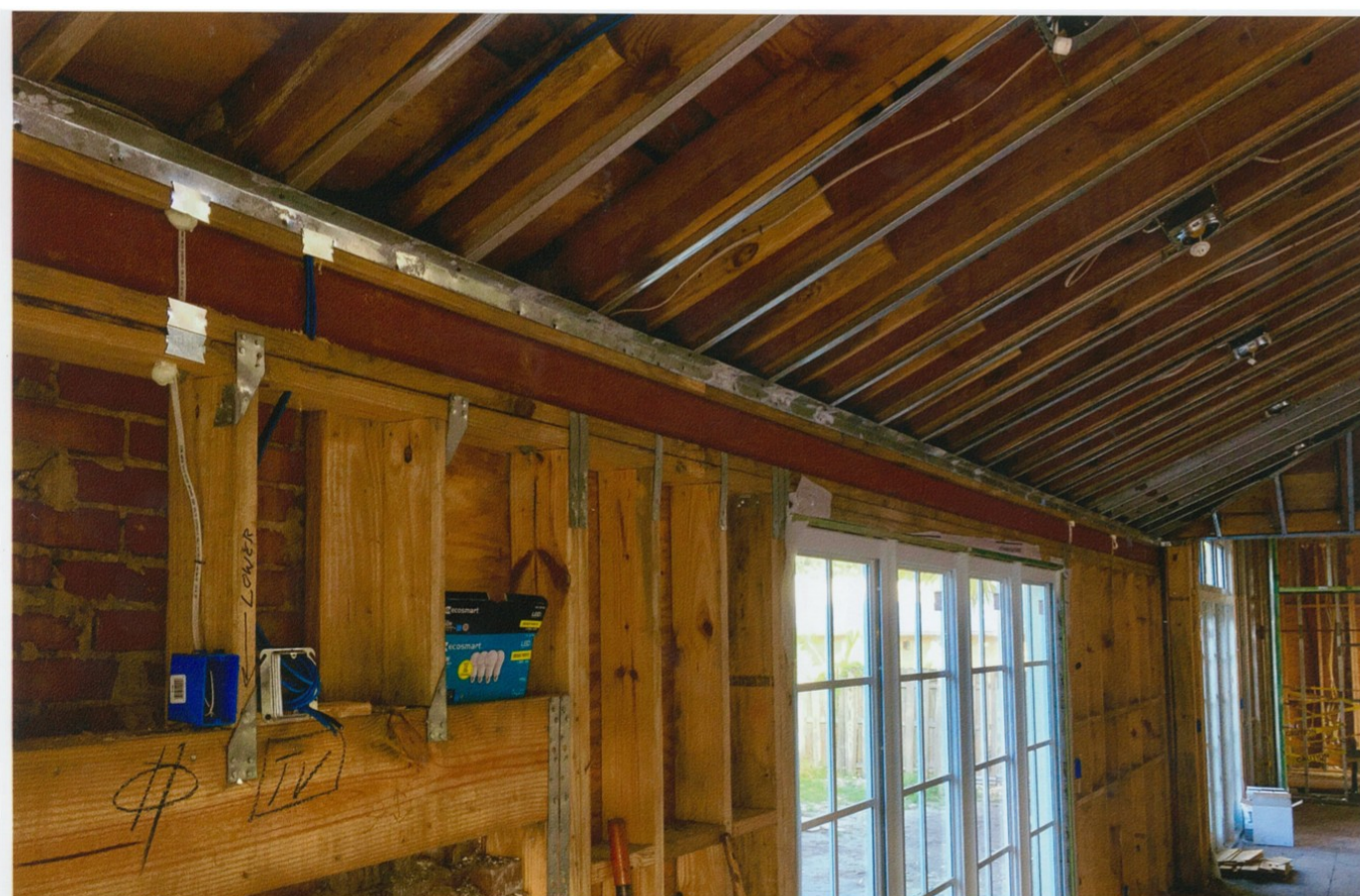
55 SE 7th Avenue- North Interior Wall- November 2016- Note Steel beam structure
