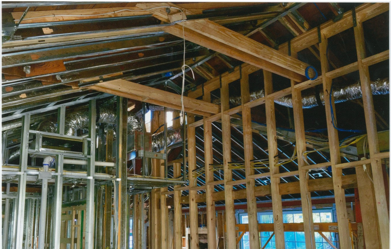
55 SE 7th Avenue- New interior framing- December 2016 Note Structural Collar Ties
