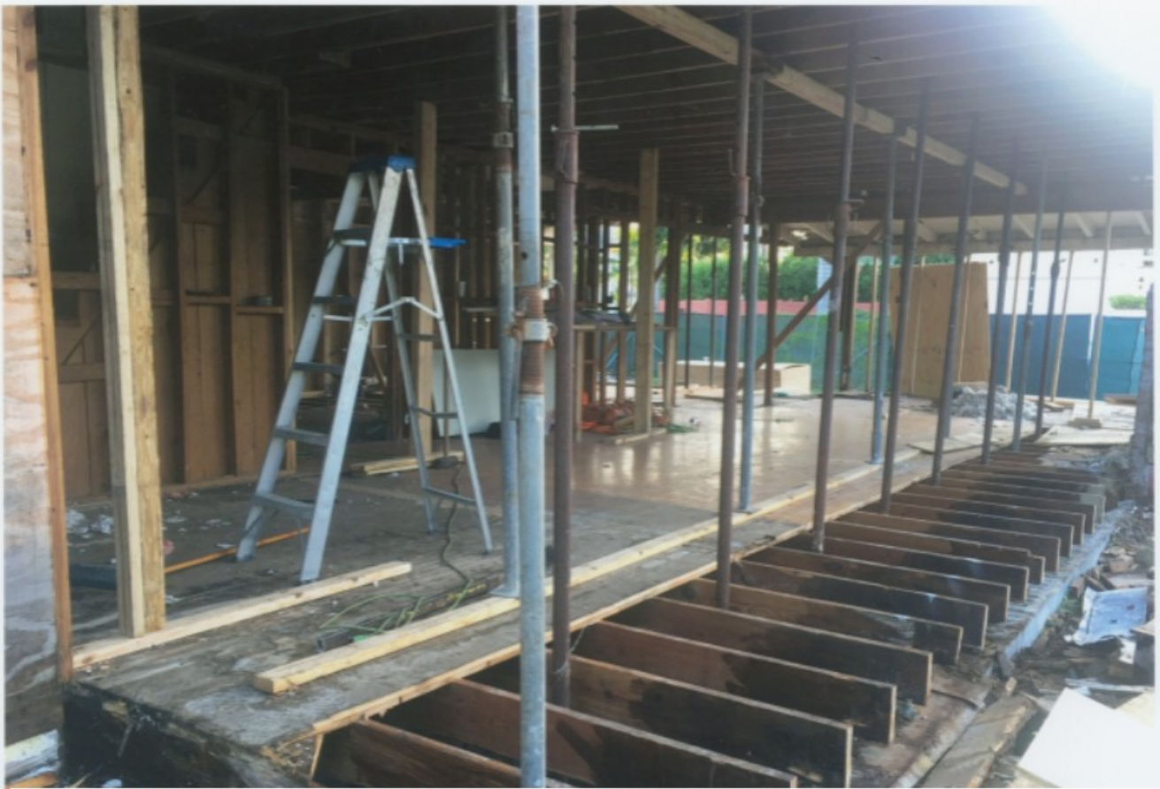
55 SE 7th Avenue-North Side original Dade County Pine floor joists revealed and retained September 2016
