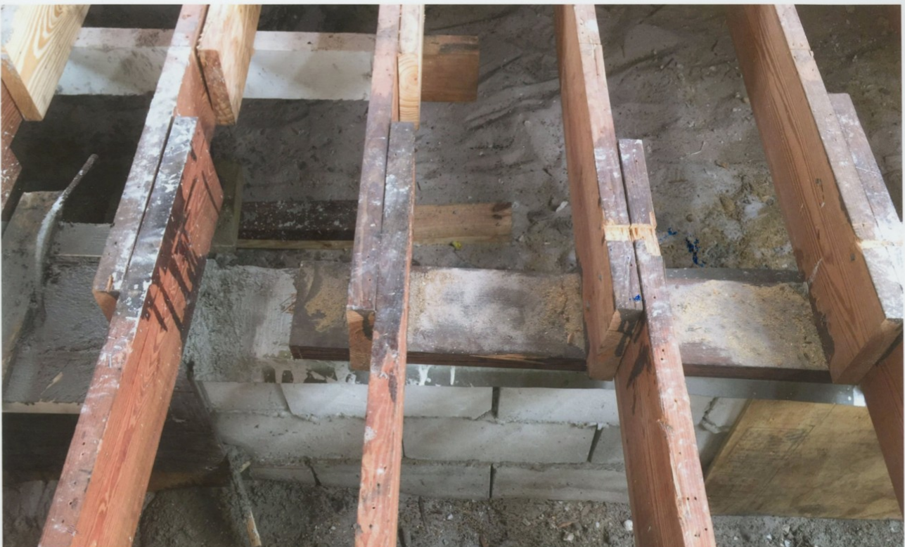
55 SE 7th Avenue- Restoration of original Dade County September 2016 Pine floor joists and concrete footing
