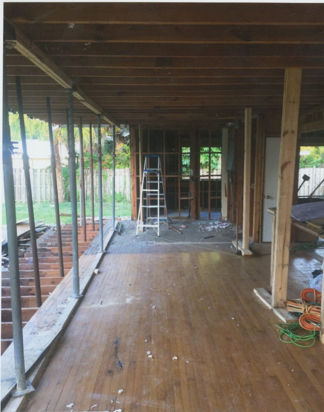
55 SE 7th Avenue- Interior North Wall- September 2016- Note Original Dade County Pine Floor Joists
