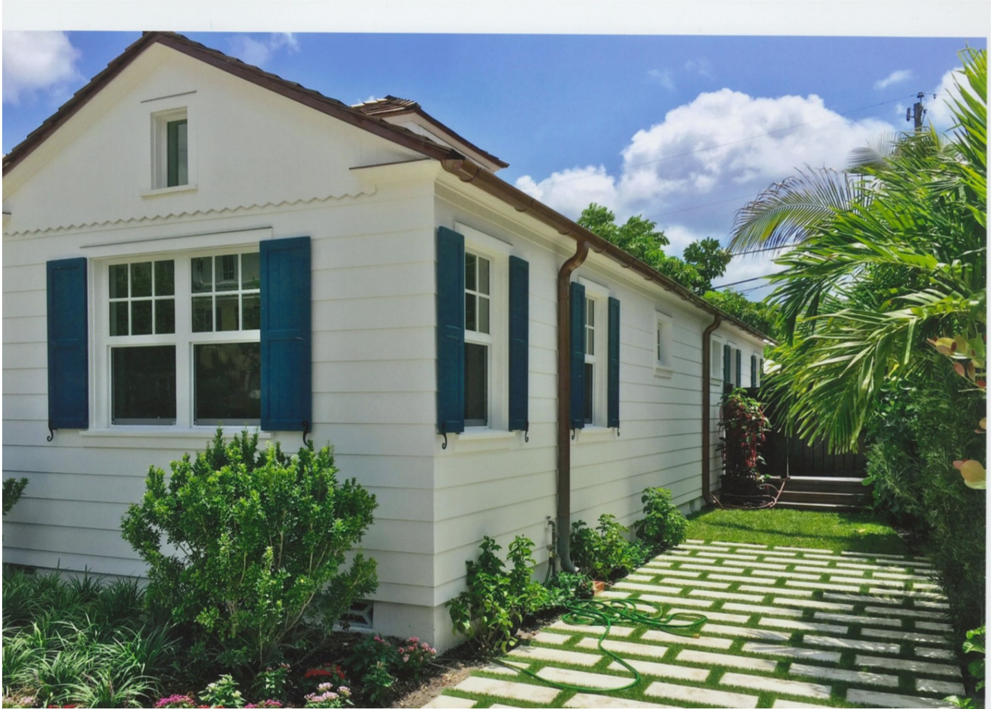
55 SE 7th Avenue- Final South Exterior-June 2017- Note Siding with Mitered Corners
