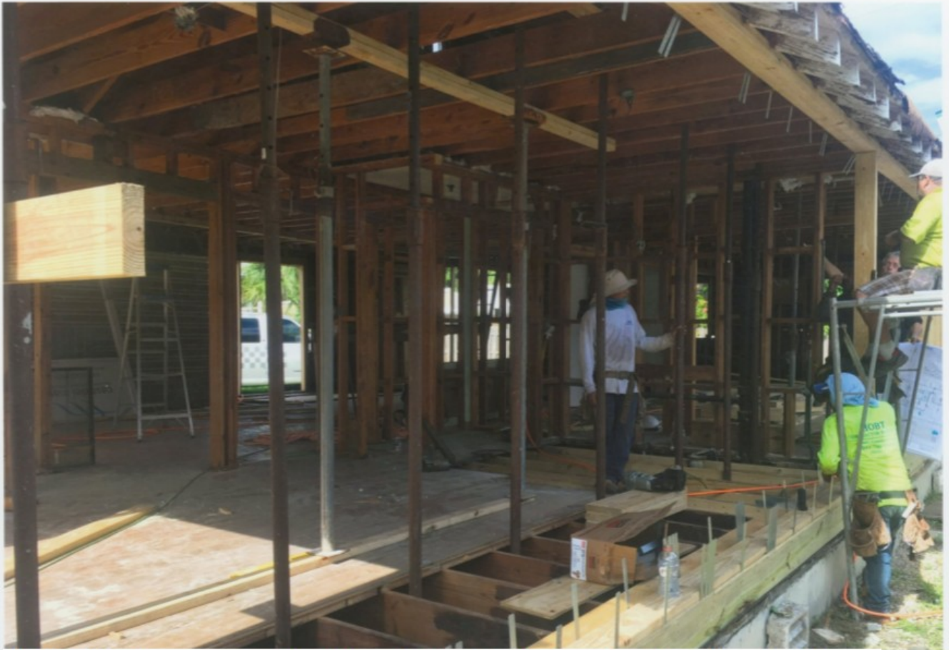
55 SE 7th Avenue- South side original Dade County Pine floor joists revealed and retained September 2016
