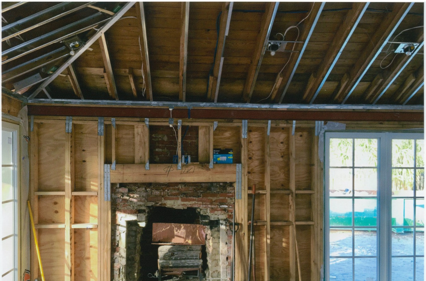
55 SE 7th Avenue- Reframe Original Fireplace November 2016 Note New structural beam
