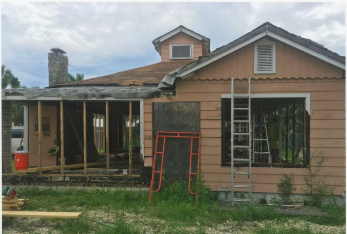
55 SE 7th Avenue- West Exterior-September 2014 Post demo of carport and reveal of original brick porch
