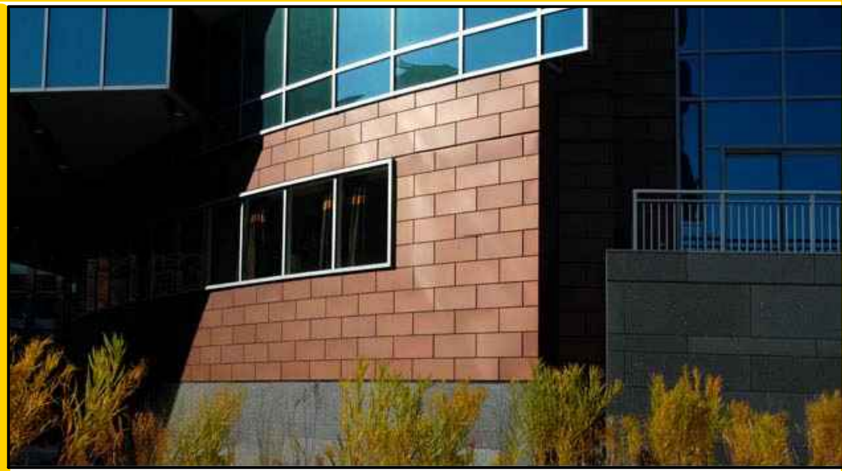
NBK TERRACOTTA 'SOLID' PANEL WALL SYSTEM
