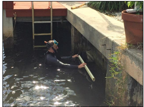
APTIM Performing Outfall Inspections - Spring 2018
