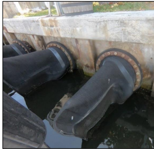
Duckbill Installed - Courtesy of APTIM 2018
