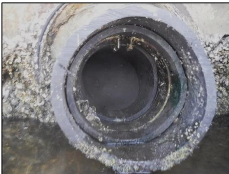
Inline Valve, Image courtesy of APTIM 2018.
