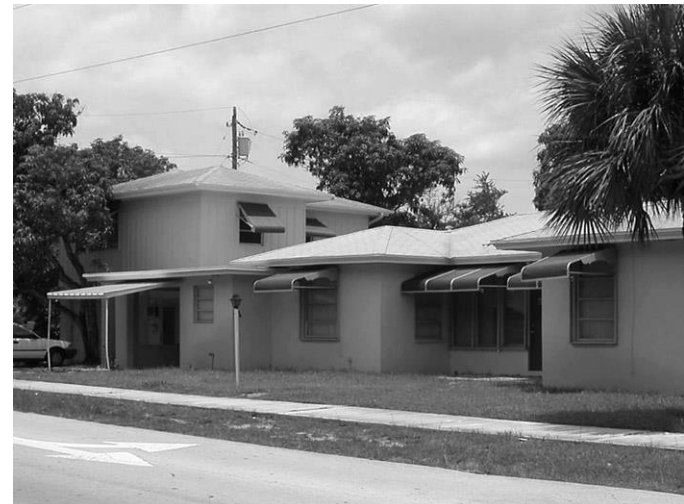
This building has stucco on the first story and wood siding on the second story.
