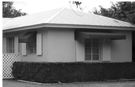
A standing seam metal, cross-hip roof
