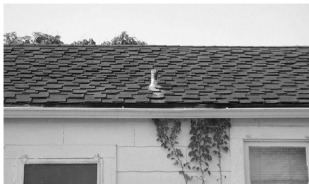
Example of irregular style roof shingles
