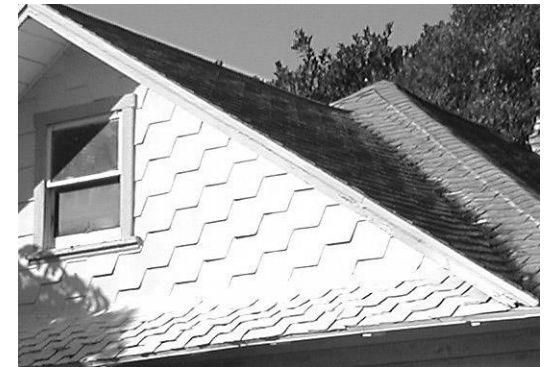
Example of hexagonal wood shingles
