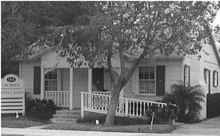
Example of a building retrofitted for access
