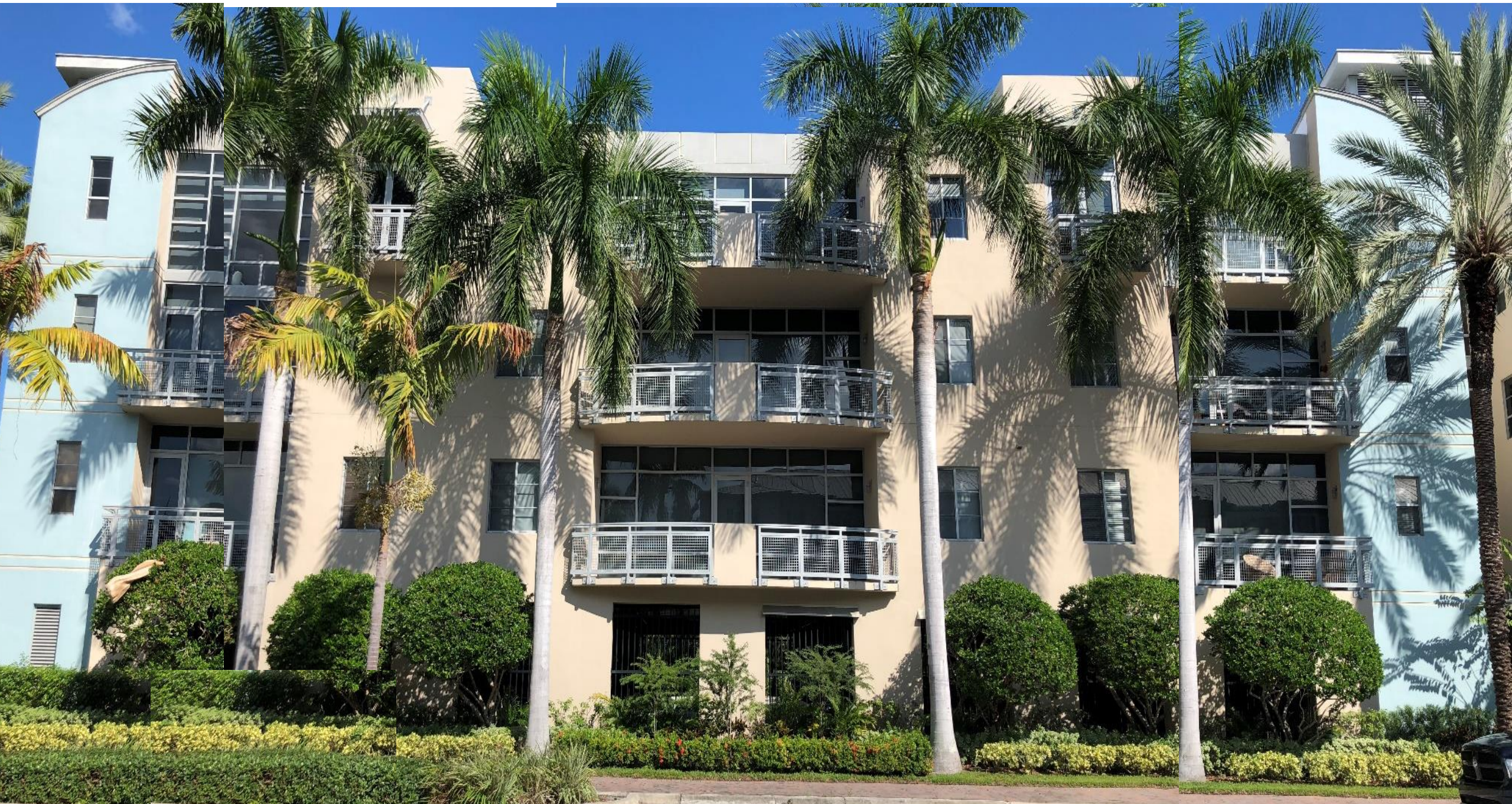
West Elevation – Half North Building
