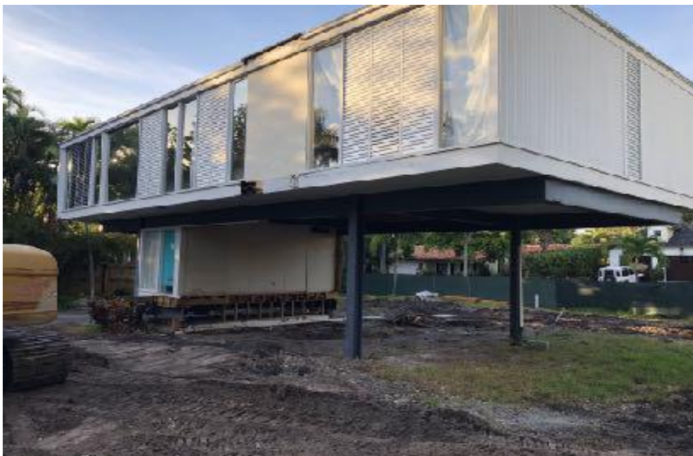
Figure 3. Post demo South view -existing 6' NAVD top of 1 st floor elevation, ground floor elevated 3' above grade, 2 nd floor elevated 12'4" above grade
