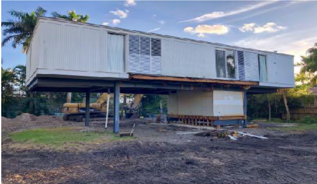
Figure 2. Post demo North view -existing 6' NAVD top of 1 st floor elevation, Ground floor elevated 3' above grade, 2 nd floor elevated 12'4" above grade
