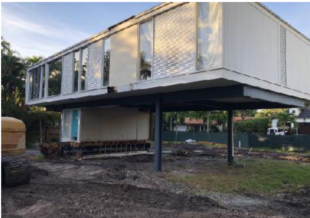
Figure 6. Post demo North view of existing 6' NAVD top of 1 st floor elevation at base of entry vestibule. Ground floor of entry vestibule is elevated 3' above existing grade, 2 nd floor structure is elevated 12'4" above existing grade.
