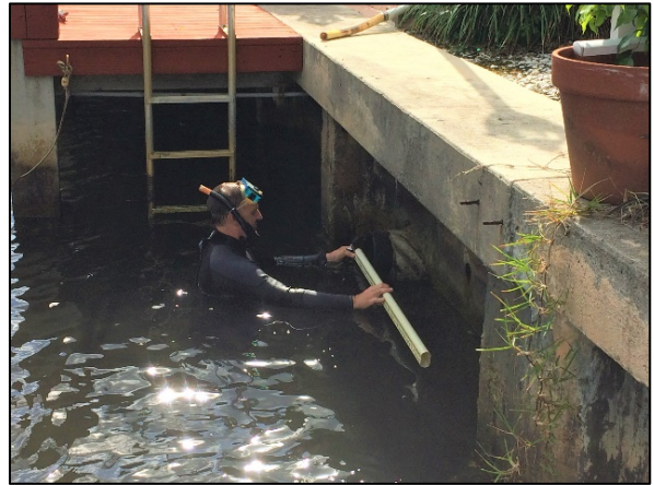
APTIM Performing Outfall Inspections - Spring 2018
