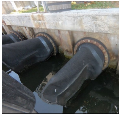
Duckbill Installed - Courtesy of APTIM 2018
