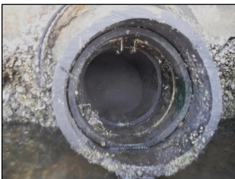
Inline Valve, Image courtesy of APTIM 2018.
