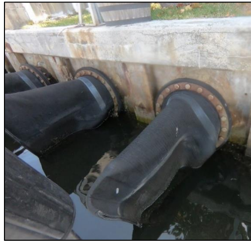
Duckbill Installed - Courtesy of APTIM 2018
