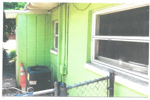
The north facade of the villa featured an add on shed to house a washing machine, a rusty chain link fence and a .cluttering tangle of conduit and wires shooting across the facade.
