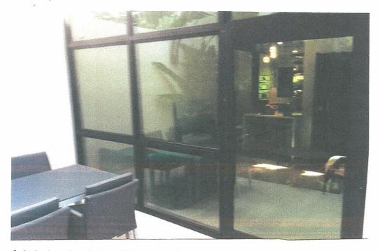
The refurbished south wall is nearly floor to ceiling commercial grade, storm-rated windows and a glass door to let as much light in as possible. The glass wall is divided in three panels, to mimic the original three panels of projected awning windows. The original outlookers remain above. The windows and door are not visible from the street.
