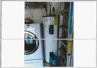
HOT WATER HEATER PIPING ATTACHED TO PRESSURE RELIEF VALVE
