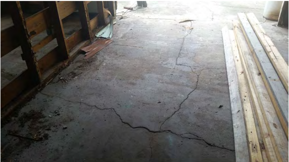
Exhibit 8. Typical Continuous Concrete slab cracks
