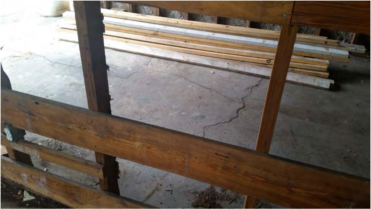
Exhibit 9. Typical Continuous Concrete slab cracks at garage area
