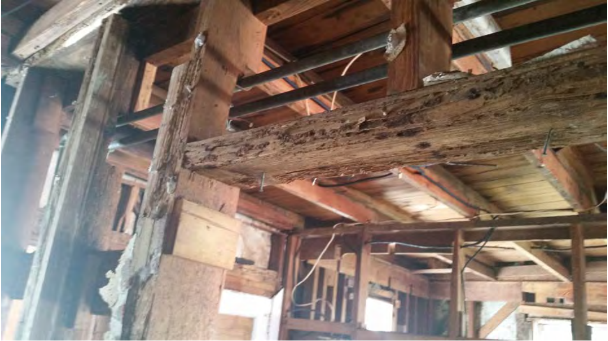
Exhibit 7. Typical rotted wood header at interior load bearing walls
