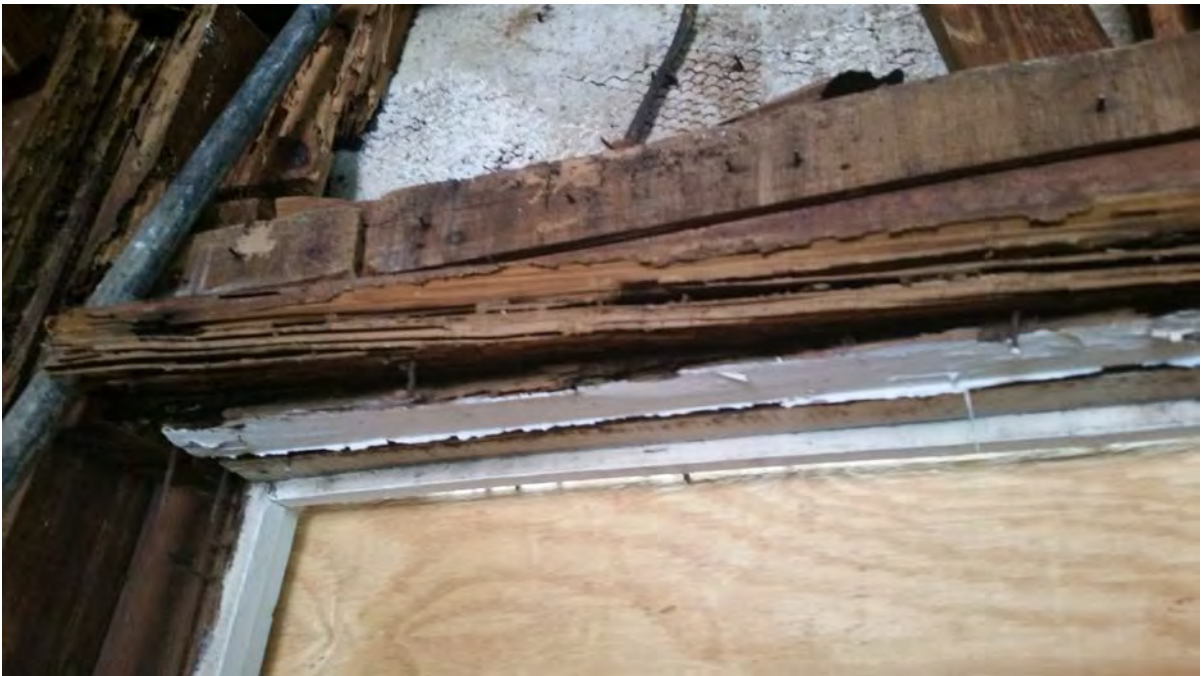
Exhibit 6. Typical rooted wood header/jamb at exterior openings
