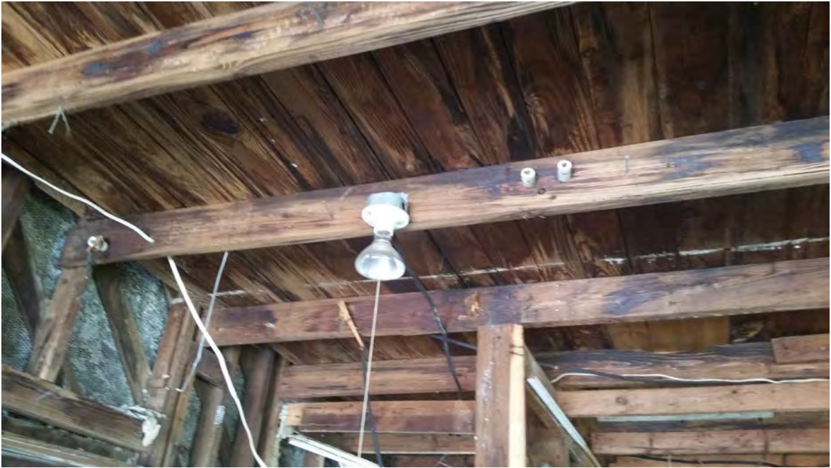
Exhibit 3. Water damaged roof joist, decking and ledger board
