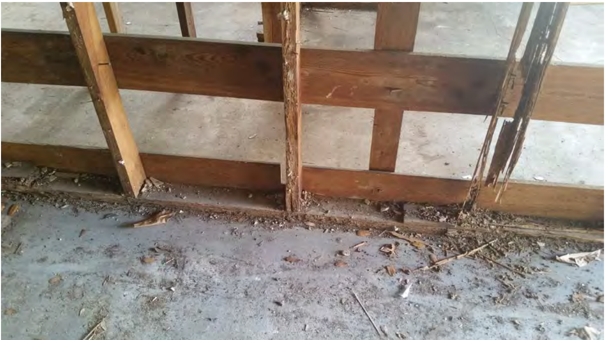
Exhibit 4. Typical missing/eroded wood wall studs
