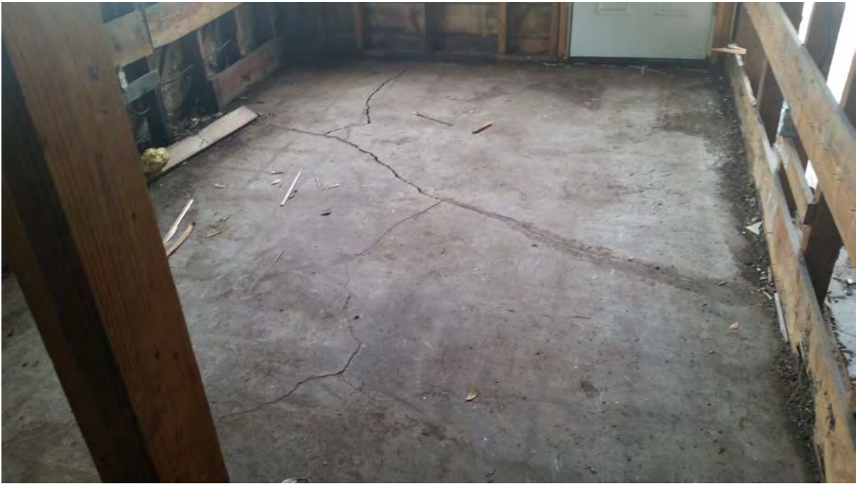
Exhibit 11. Typical Continuous Concrete slab cracks at room
