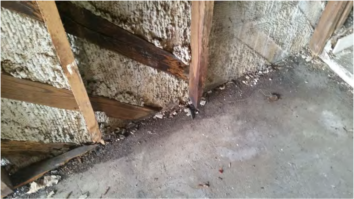
Exhibit 5. Typical Missing/eroded base plate of exterior wood frame walls
