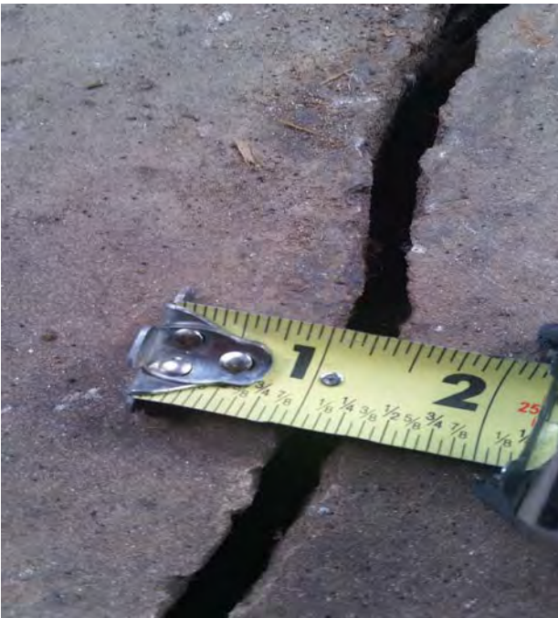
Exhibit 12. Typical Crack separation
