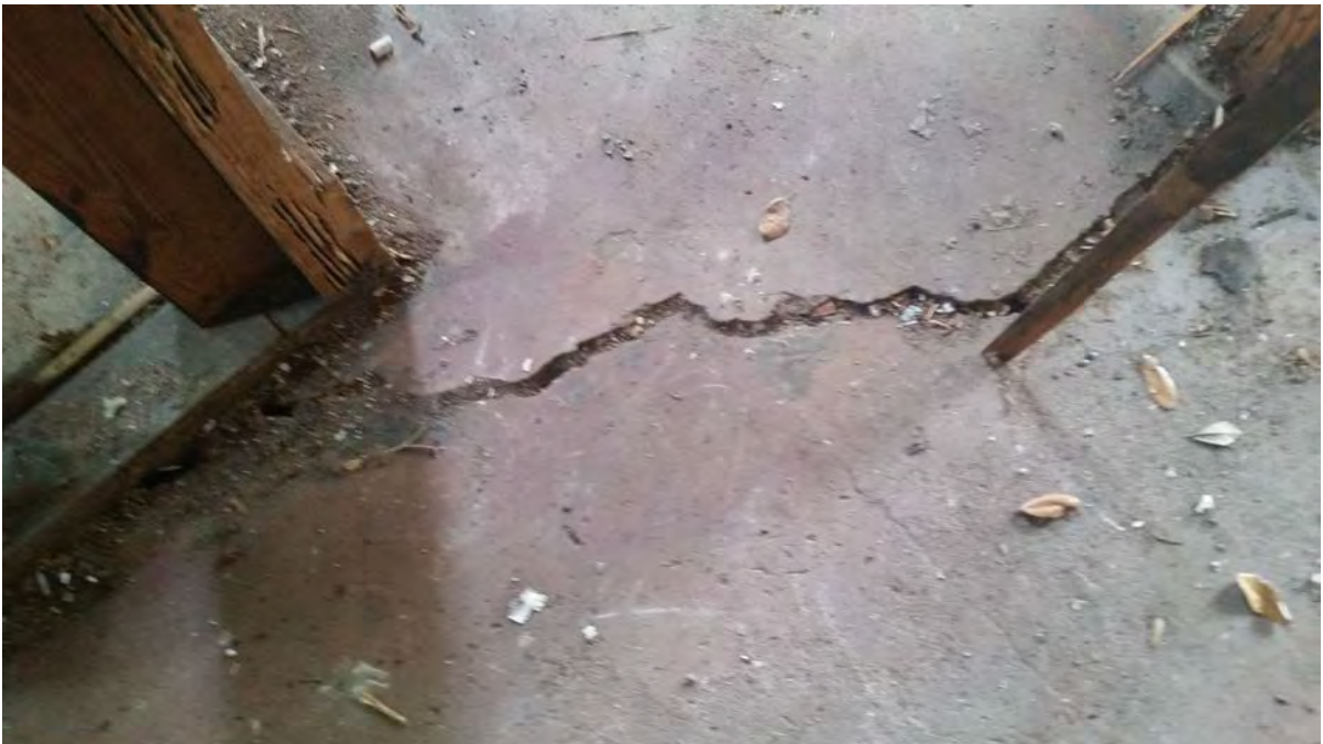
Exhibit 10. Typical Continuous Concrete slab cracks
