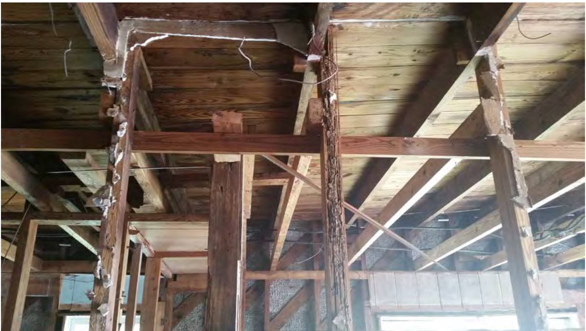
Exhibit 2. Typical Rotted Wood Wall Studs
