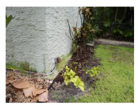
GARAGE FLOOR SLAB EXTENDS OUTSIDE FRAME WALL – DETAIL OF THIS "LEDGE" PERMITS WATER-DAMAGE TO THE EXISTING SILL-PLATE AND STUDS (SUGGEST REPLACEMENT WITH MASONRY OF CONCRETE TO PREVENT FUTURE DAMAGE)
