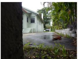
EXISTING GARAGE IS AT LOW-POINT OF LOT – PAVED DRIVEWAY DIRECTS RAIN WATER TO FRONT OF STRUCTURE – PROPOSE SETTING REPLACEMENT STRUCTURE 4" MINIMUM (HIGHER) TO DIRECT SURFACE FLOW AROUND PROPOSED MASONRY STRUCTURE.
