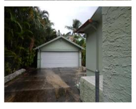
VIEW OF EXISTING WOOD-STUCCO GARAGE. (HISTORIC DETAIL LIMITED TO SMALL "CORBEL") – METAL DOOR & STUCCO TRIM-DETAIL ADDED, ASSUME AT TIME OF FRAMING REPAIR? STRUCTURE SHOULD BE REPLACED WITH ONE SUITABLE FOR THE OCCASIONAL SUBMERSION WITHOUT STRUCTURE IMPACT – WOOD IS NOT ACCEPTABLE.
