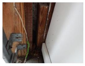
ALL WOOD STUDS (IN-THIS-EXPOSED-VIEW) ARE "NON-ORIGINAL" ALL EXISTING (HISTORIC) FRAMING HAS BEEN REPLACED – TYPICAL AT EXPOSED LOCATIONS.
