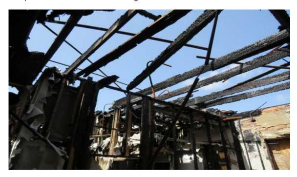
The interior wood framed walls were severely charred and there was a significant amount of debris on the floor in the south section of the building.
