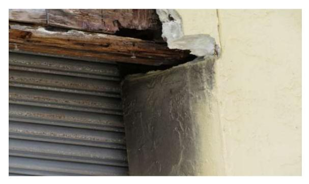
The brick parapet wall was broken on the east side of the building.
