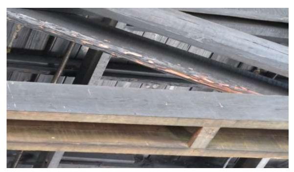
The southernmost steel truss above the north section of the building was warped.
