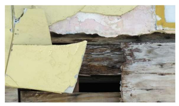
There were cracks in the stucco at the northeast corner of the building.
