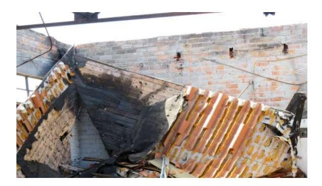
A portion of the roof framing remained in place above the north section of the building. The remaining roof framing was covered in soot and partially charred.
