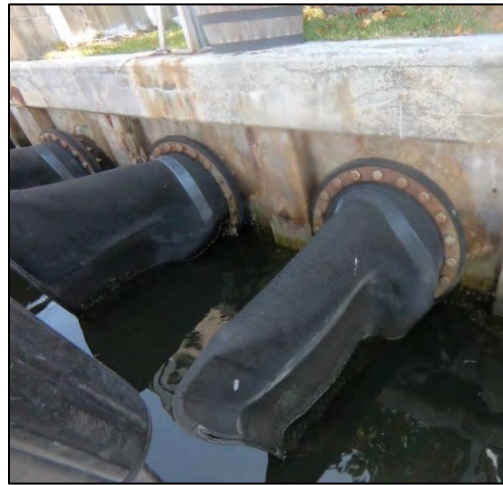
Duckbill Installed - Courtesy of APTIM 2018
