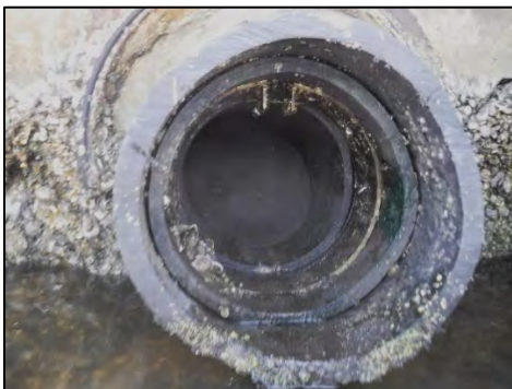
Inline Valve, Image courtesy of APTIM 2018.
