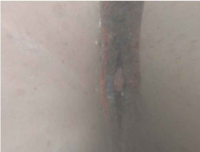
Marine Way E 2. Duckbill does not seal.
