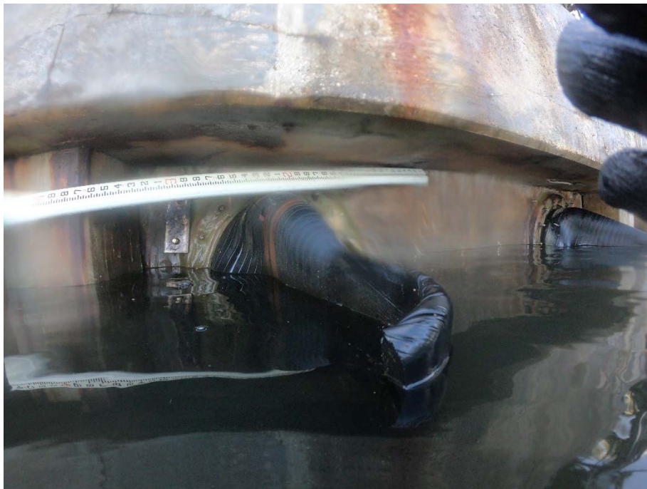
Venetian Drive W 2. A few barnacles were present inside, but the valve did seal. No oysters were present on the seawall.
