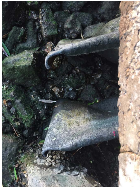
Beach Drive S 1 & Beach Drive S 2. Seals but duckbill rests in sediment.
