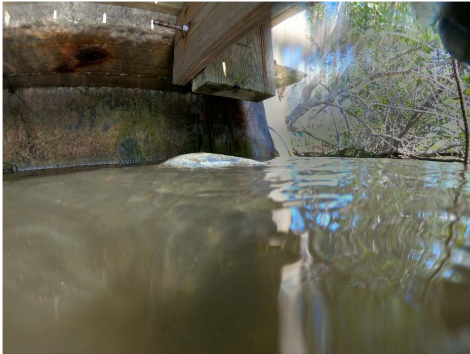
SE1st Street E 3. Barnacles inside of duckbill prevent closure.
