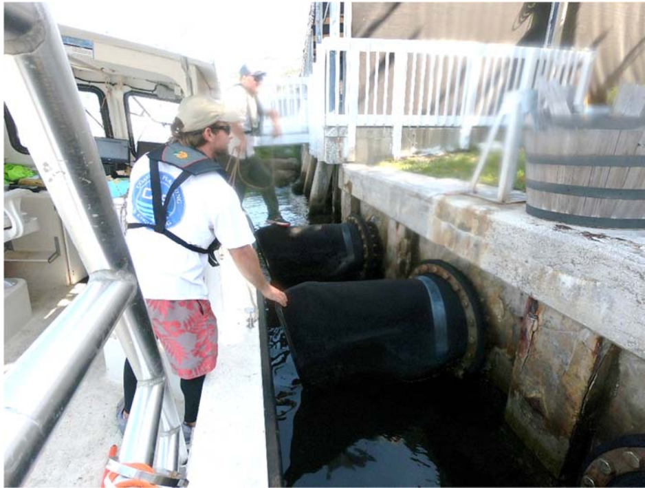
MacFarlane Drive W 6. Barnacles in the bottom of the duckbill may prevent full closure.
