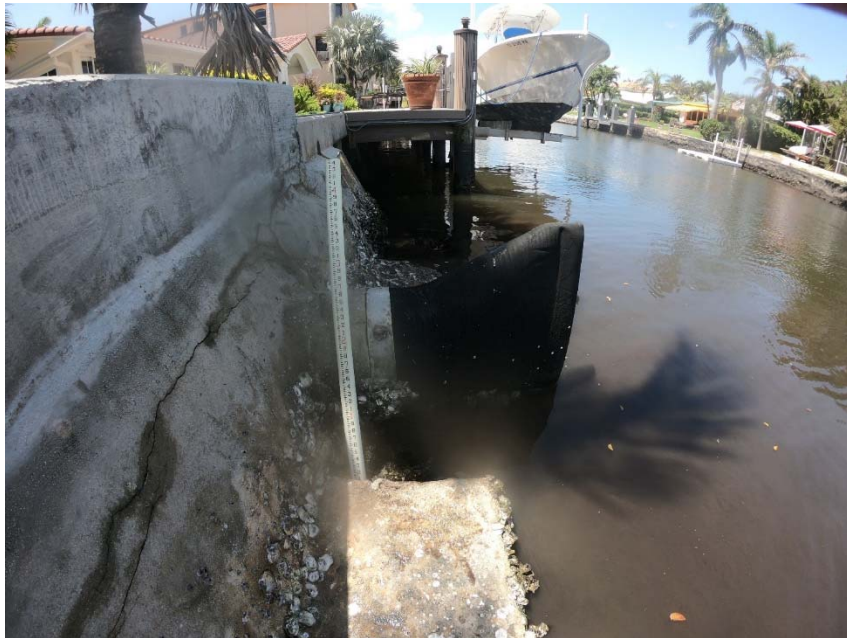
Rhodes Villa Ave N2. Clean due to high invert elevation.
