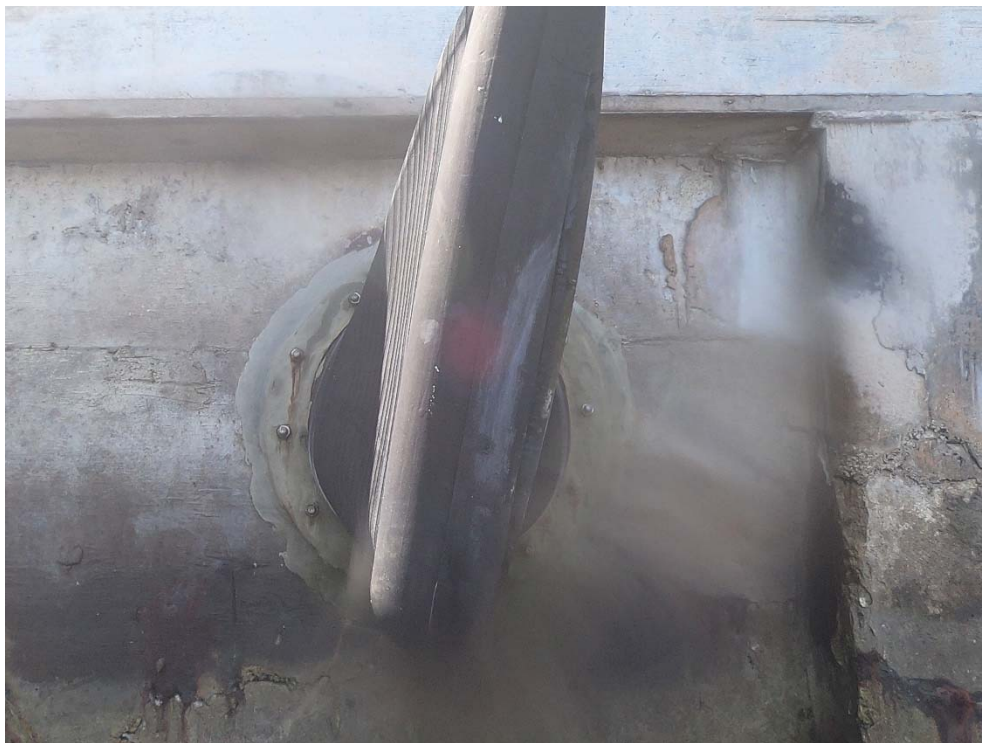
Basin Drive N 1. Duckbill is above MHW. Clean due to high invert elevation.
