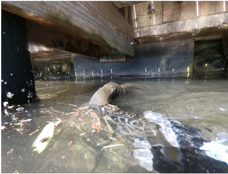
SE 1 st Street E 1. Barnacles inside of duckbill prevent closure.
