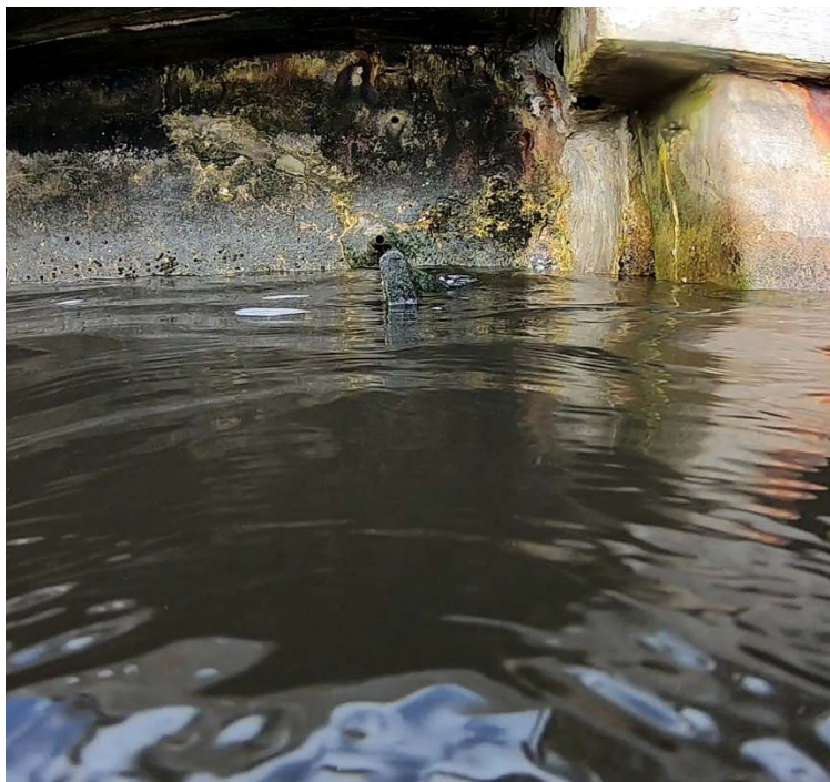
Cypress Drive E. Oysters are in the bottom of the duckbill preventing closure.
