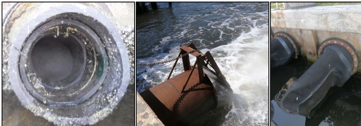
Figure 15. Examples of Functioning Backflow Prevention Devices Currently Installed (left: inline valve, center: flap gate, right: recurved duckbill valve).
