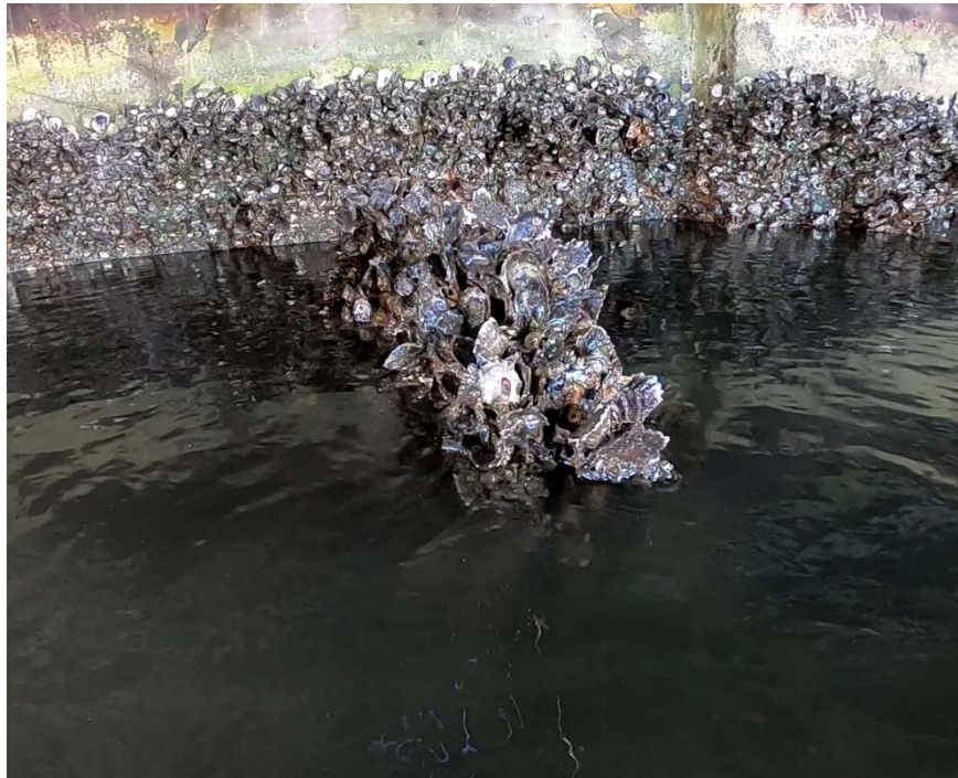
Spanish Circle N. Oysters are in the bottom of the duckbill preventing closure.
