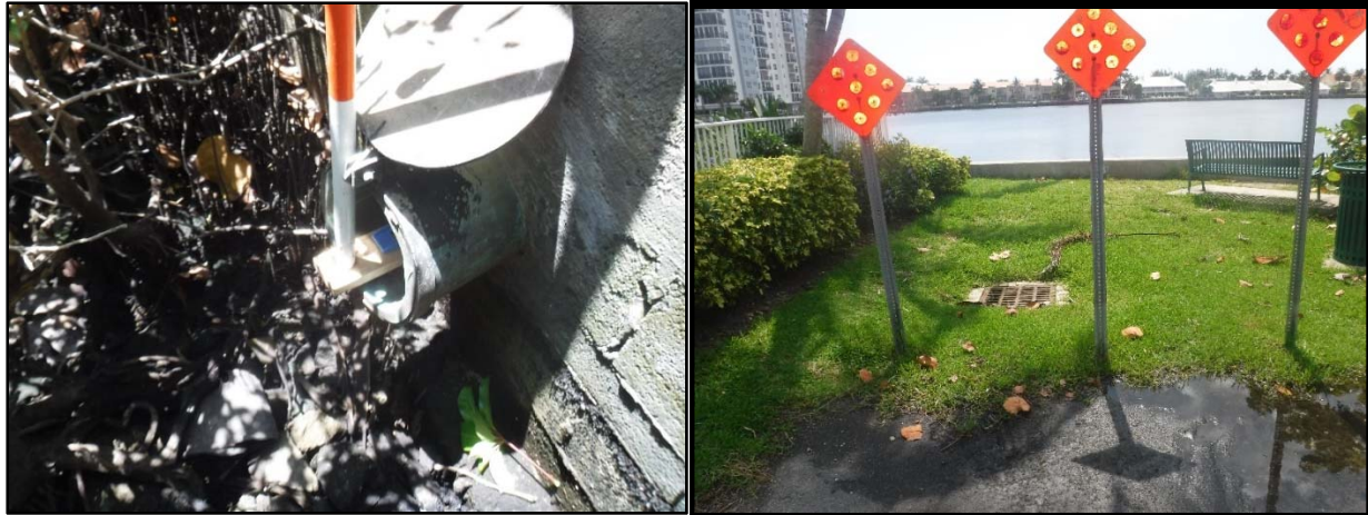
Figure 11. Surveying the Invert Elevation for an Outfall Pipe Located Along Marine Way (left). Example of a Stormwater Inlet Upstream of a Discharge at SE 3 rd Street (right).
