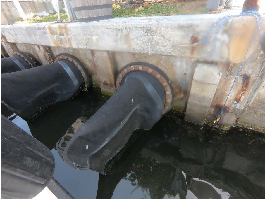
MacFarlane Drive W 4. Barnacles in the bottom of the duckbill may prevent full closure.
